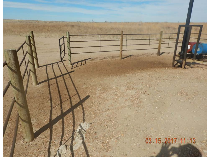
Photo 2: Stained soil at exhaust
