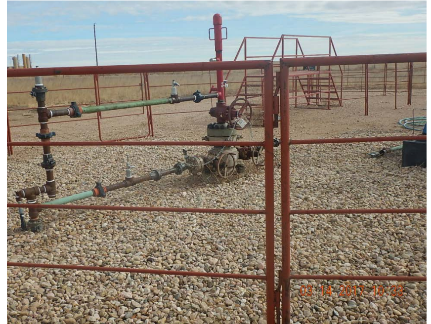
Photo 2: Wellhead looking NE
