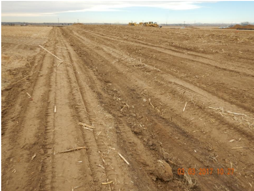
Photo 5. Photo taken from the eastern location, facing South. Ditch and berm BMP installed around perimeter of location. Also, topsoil stockpile stored along eastern perimeter of location.
