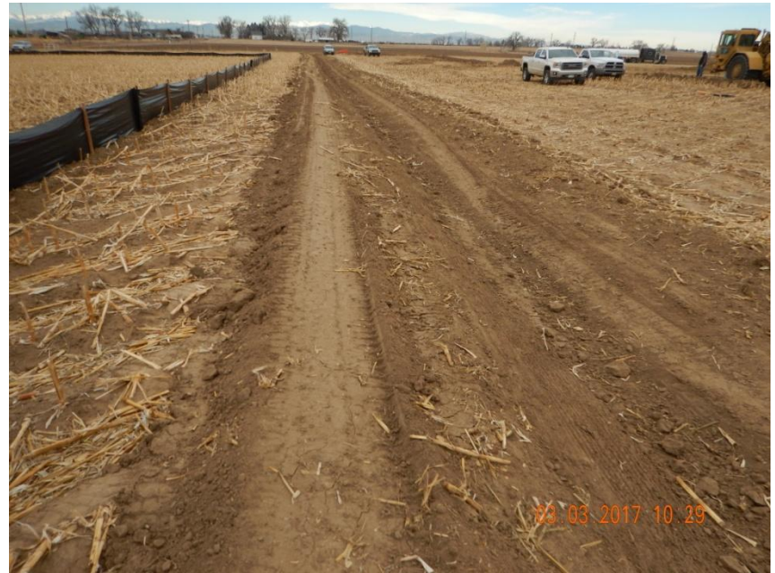
Photo 6. Photo taken from the southern location, facing West. Ditch and berm BMP installed around perimeter of location. Location with silt fence to the south is not part of this location or Operator.
