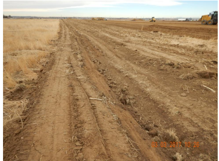
Photo 4. Photo taken from the eastern location, facing South. Ditch and berm BMP installed around perimeter of location.
