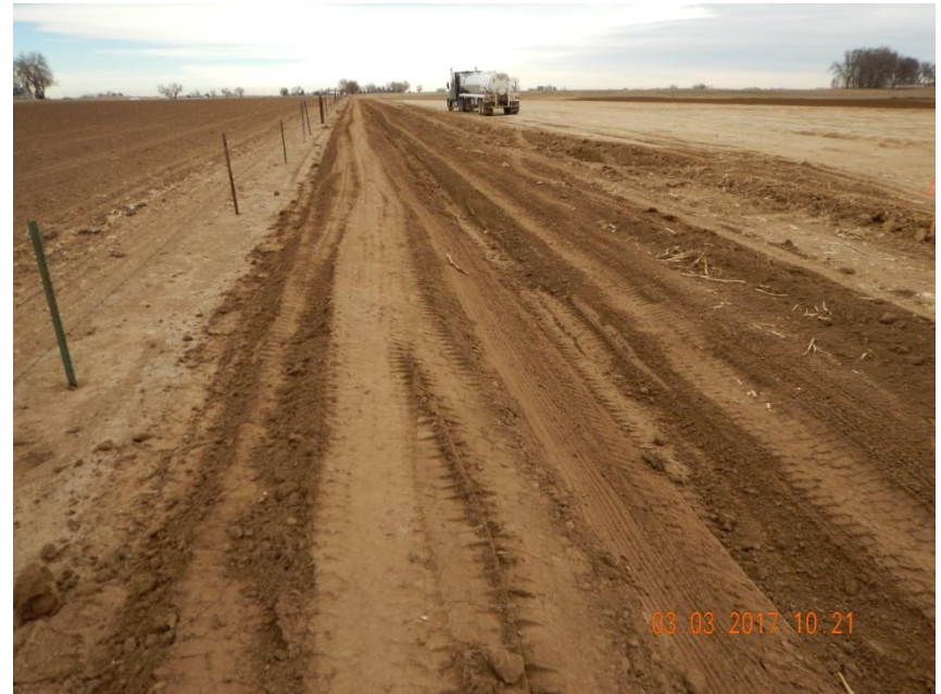
Photo 2. Photo taken from the western location, facing North. Ditch and berm BMP installed around perimeter of location.
