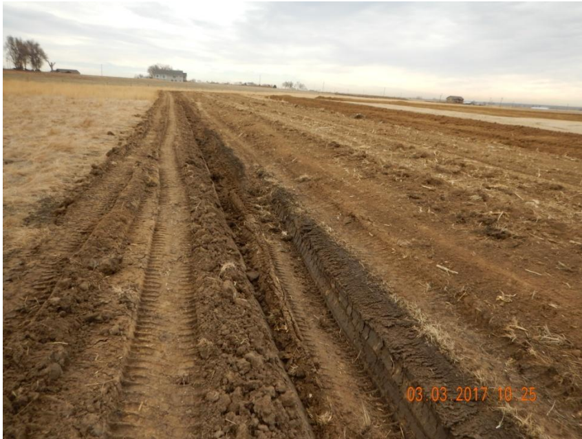
Photo 3. Photo taken from the northern location, facing East. Ditch and berm BMP installed around perimeter of location. Ensure berm BMPs are consistently compacted throughout location.
