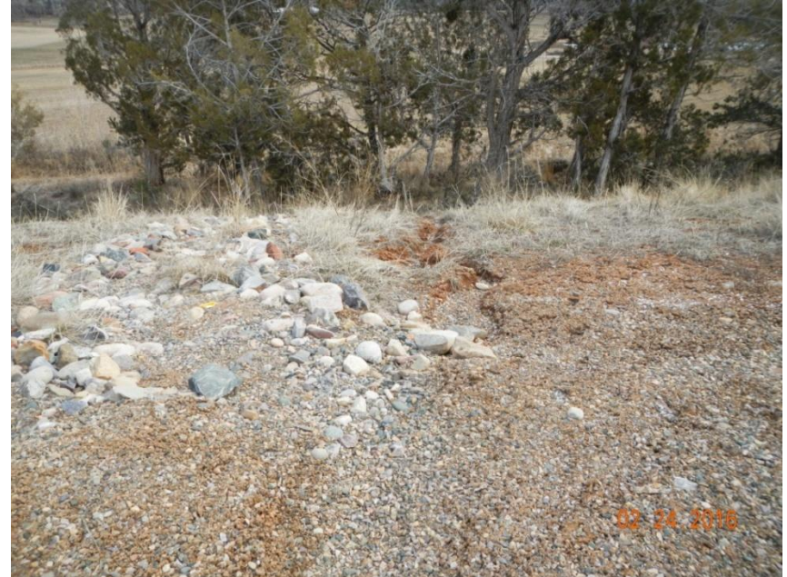
Photo 4: View of erosion occurring around cobble run-down in the eastern portion of the project area.
