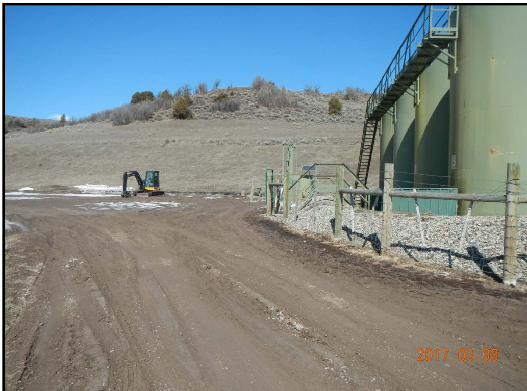
Tank Battery (4 tanks) Earthen Berm
