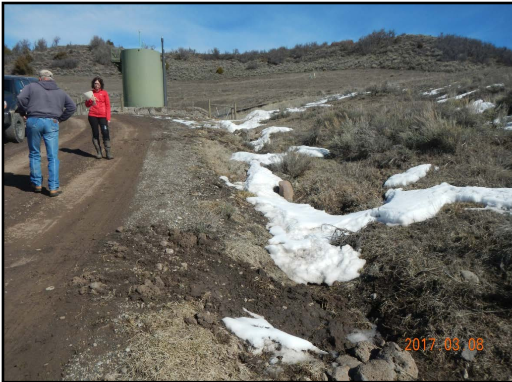
Roadside ditch with snow melt. Rock check dams to control velocity, erosion and sediments. SG environmental consultant took soil samples near the tank battery, at a location down on the side ditch (bottom of photo), and halfway (up-gradient of where people are standing).
