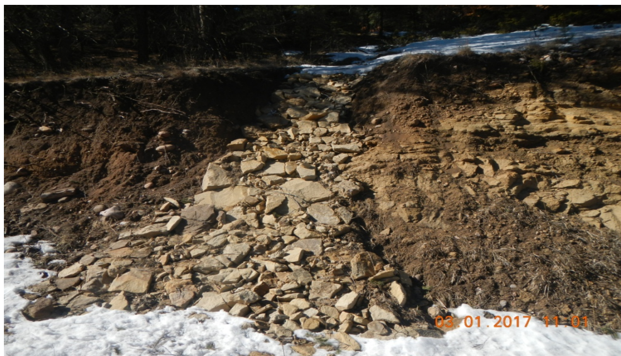
photo 6: Rock rip/rap placed along the cut slope of the road.
