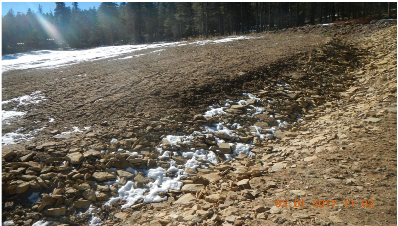
photo 10: Rock rip/rap placed along the diversion ditch.
