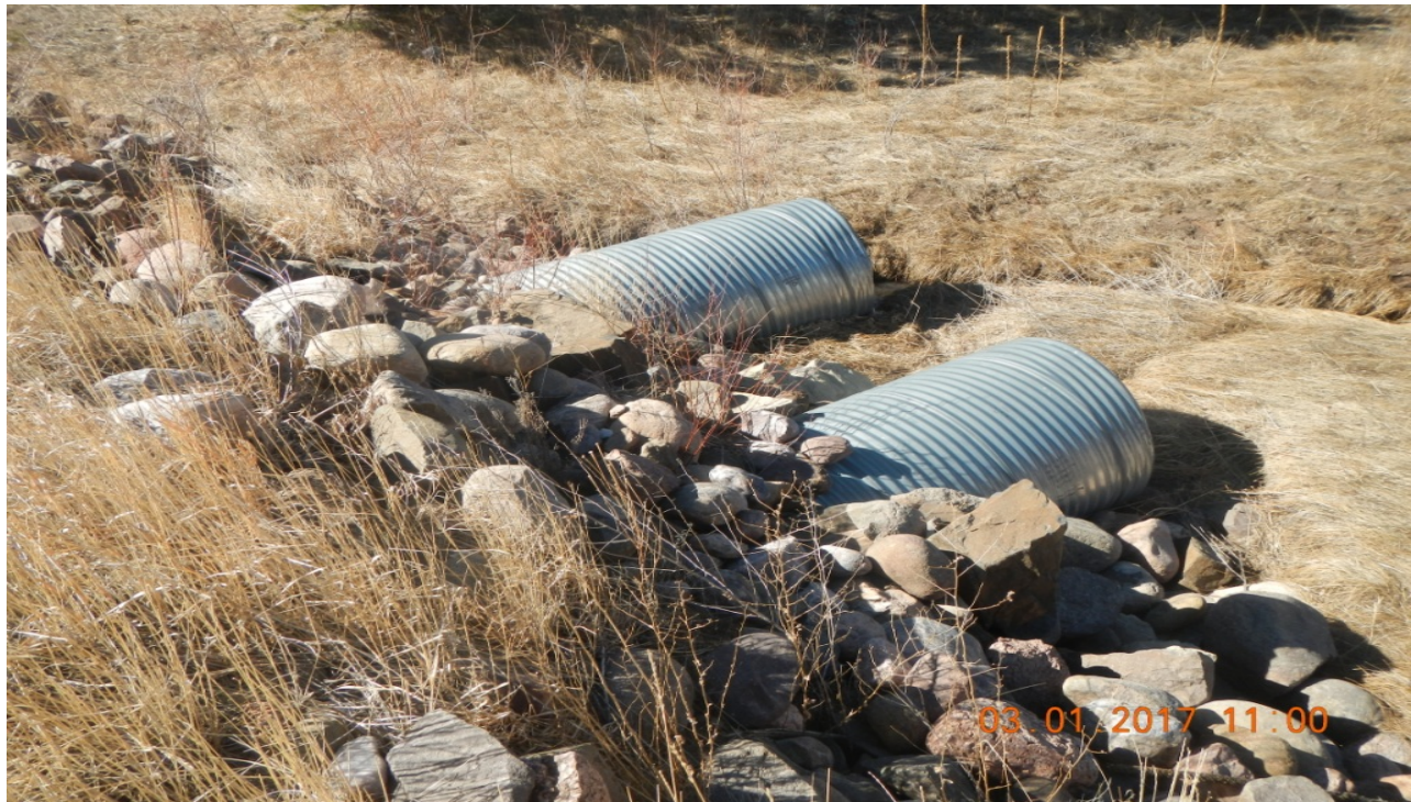
photo 3: The culverts installed along the road for the intermittent creek.
