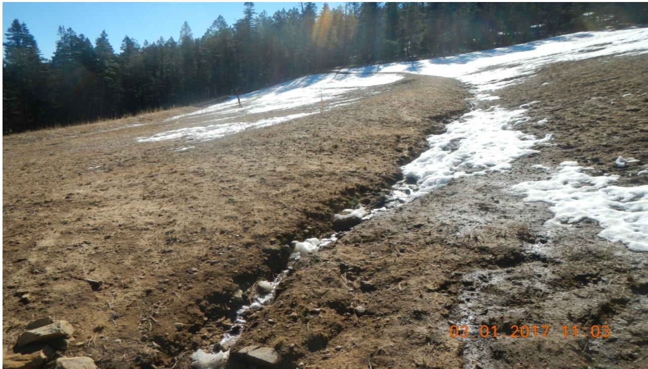
photo 11: A diversion ditch is installed along the contour of the slope.
