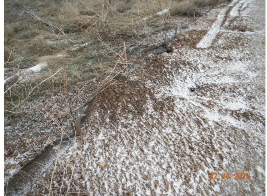
Photo 4: View of sediment over-topping wattles in the eastern portion of the project area.
