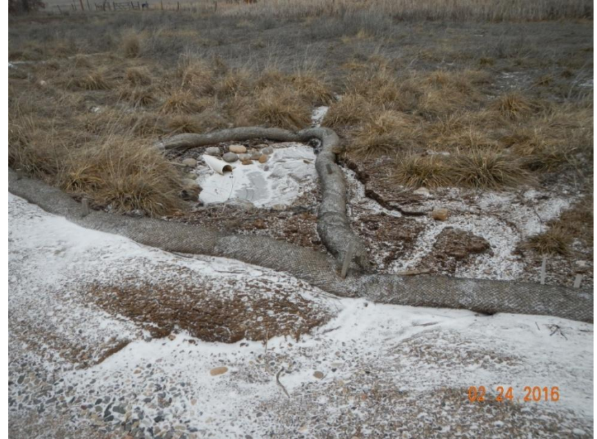
Photo 6: View of another area where stormwater flows beneath the wattles in the eastern portion of the project area.
