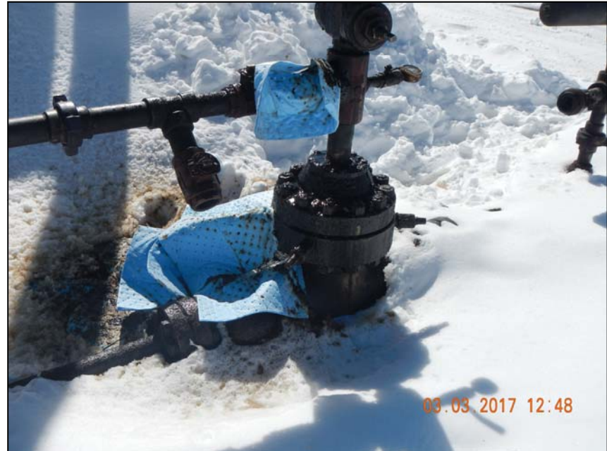
Photo 5. Close up of ongoing release at wellhead.
