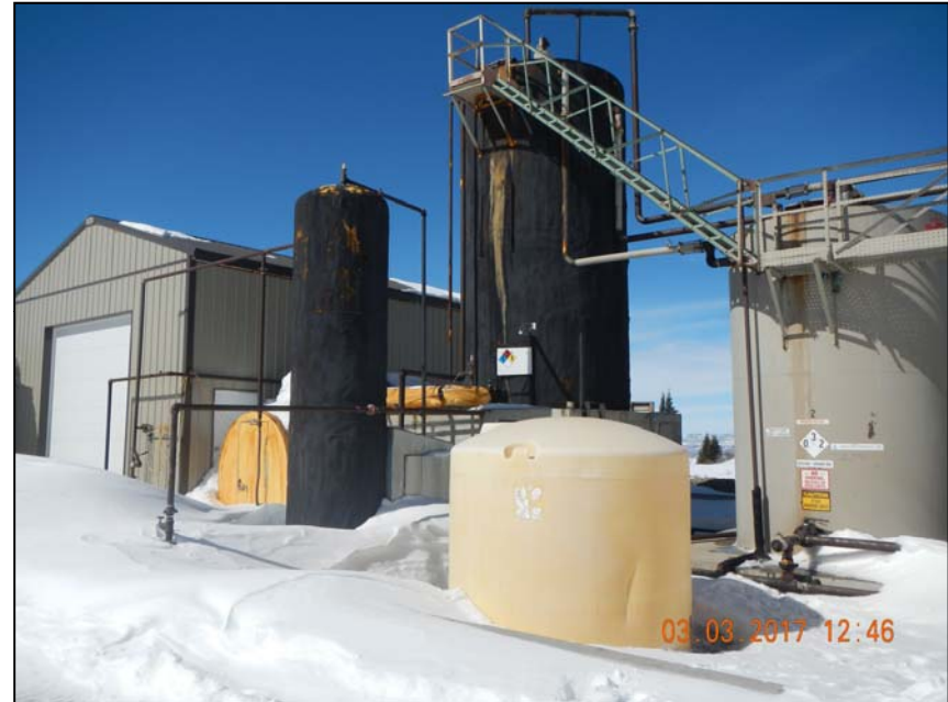
Photo 3. Missing tank labels.
