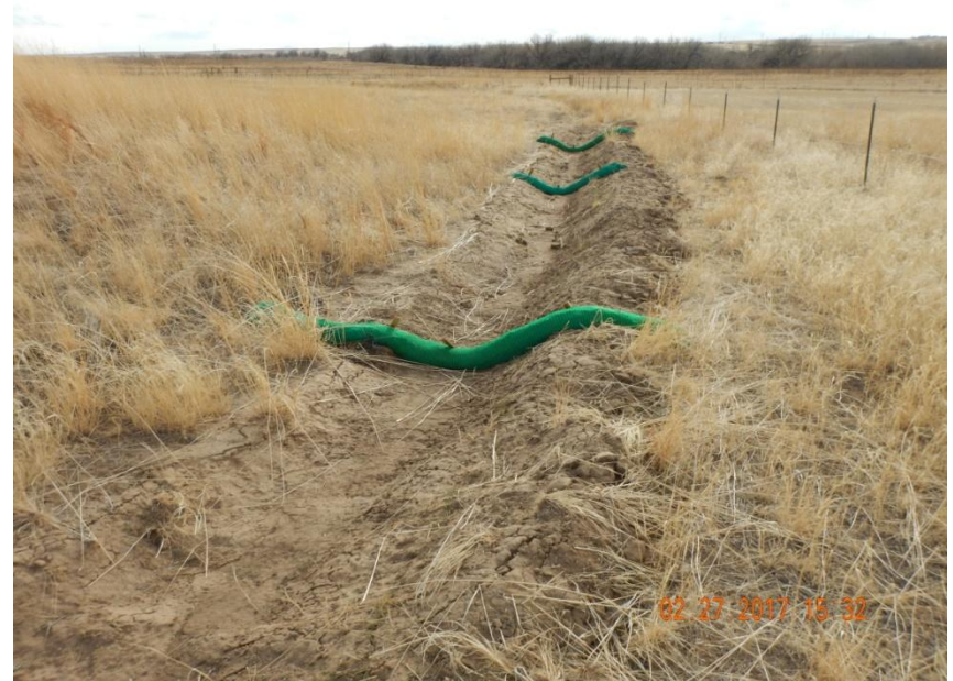
Photo 10. Photo taken from the northwest location along the current interim area, facing South. Wattles installed throughout the ditch BMP area.
