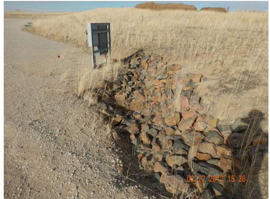
Photo 4. Photo taken from entrance of location along the current interim area, facing North. Culvert installed with rip rap as inlet protection.
