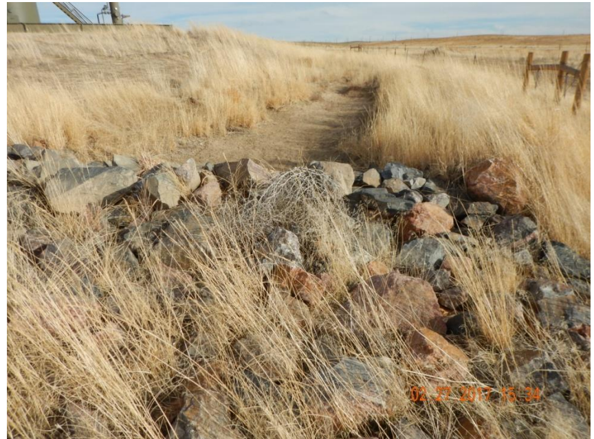
Photo 12. Photo taken from the southwest location along the current interim area, facing Southeast. Sediment trap installed with armored outlet protection. Did not observe any sediment discharge at the sediment trap location.
