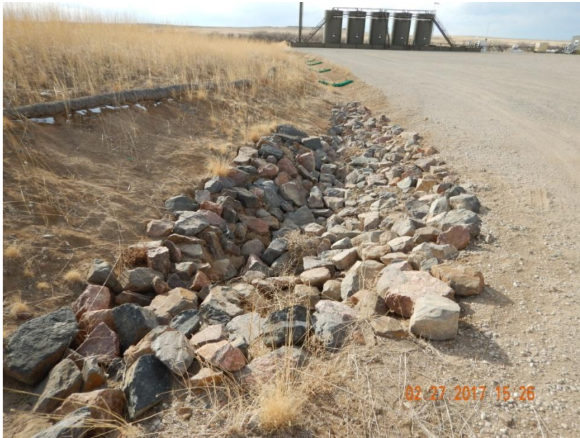
Photo 3. Photo taken from entrance of location along the current interim area, facing Northwest, towards the production area. Rip rap and wattles installed along the interim area and ditch BMP area.
