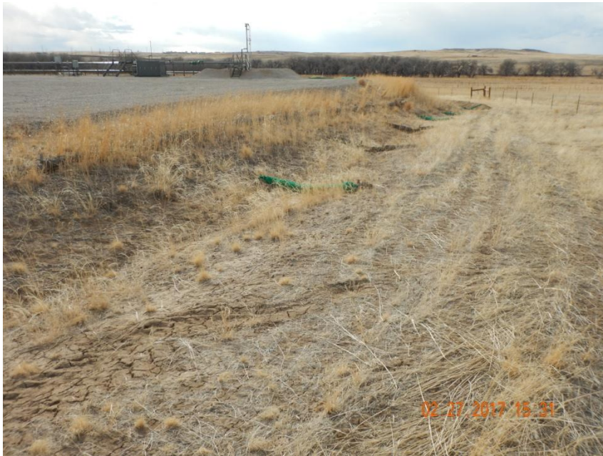
Photo 9. Photo taken from the northern location along the current interim area, facing West. Wattles installed throughout the ditch BMP area.
