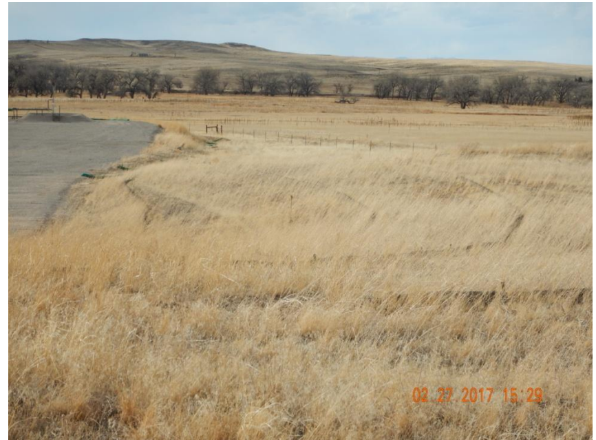
Photo 6. Photo taken from the northeast location along the current interim area, facing West. Wattles installed throughout the interim, south-facing slope area.
