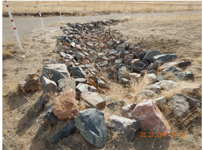
Photo 2. Photo taken from entrance of location, facing Southwest. Culvert installed with rip rap as outlet protection.
