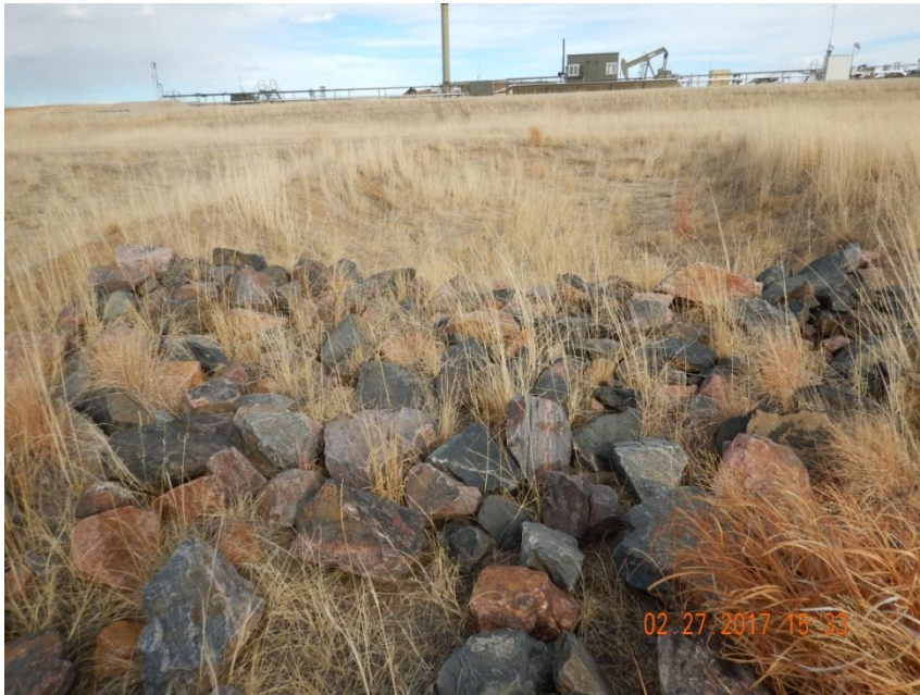
Photo 11. Photo taken from the western location along the current interim area, facing East. Sediment trap installed with armored outlet protection. Did not observe any sediment discharge at the sediment trap location.
