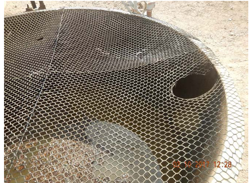
Photo 3: Hole in netting unrepaired
