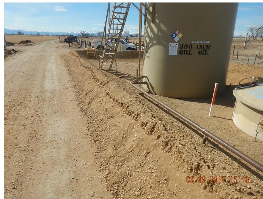
Photo 2: Berms at tank battery have been repaired.
