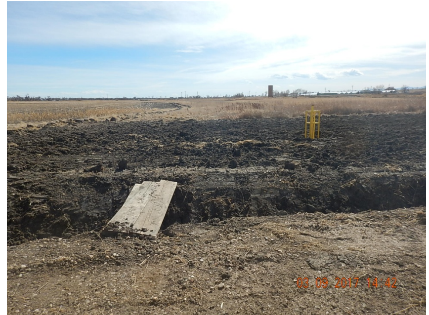
Photo 2: meter run removed, area ripped
