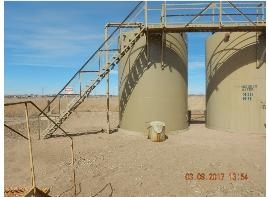
Photo 5: No labels on production tank
