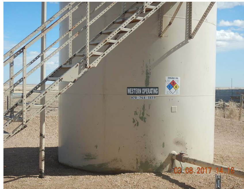
Photo 2: No capacity on production tank
