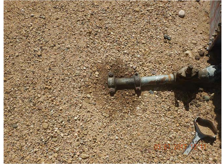
Photo 3: Stained soil at valve
