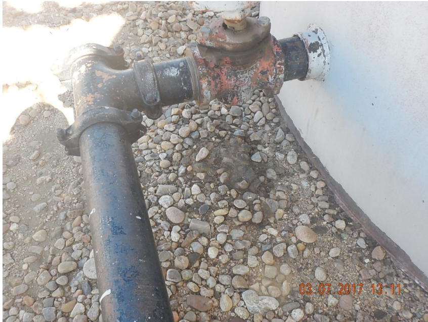
Photo 5: Stained soil beneath loadout
