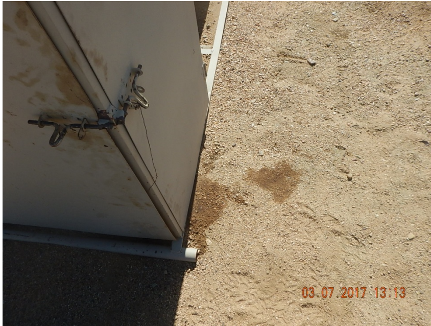
Photo 7: Stained soil at separator
