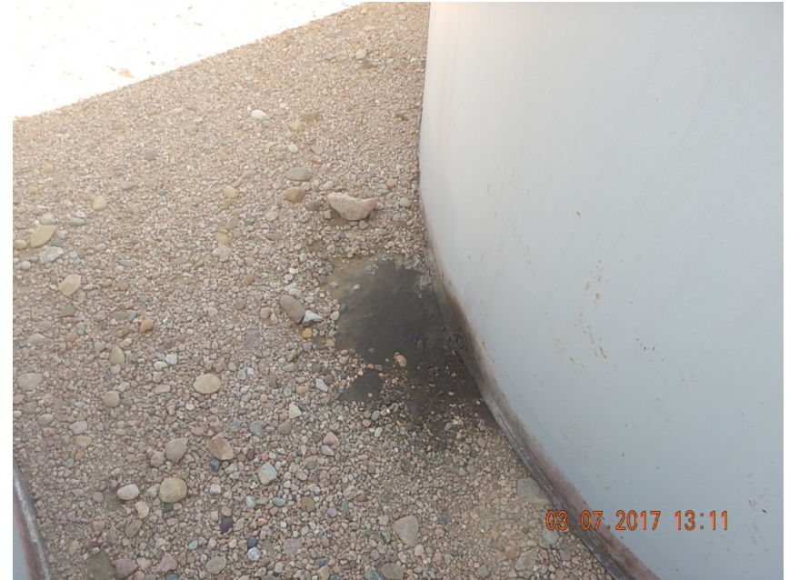
Photo 6: Stained soil at tank
