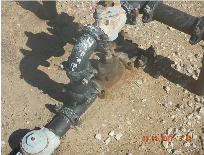
Photo 3: Stained soil at fitting
