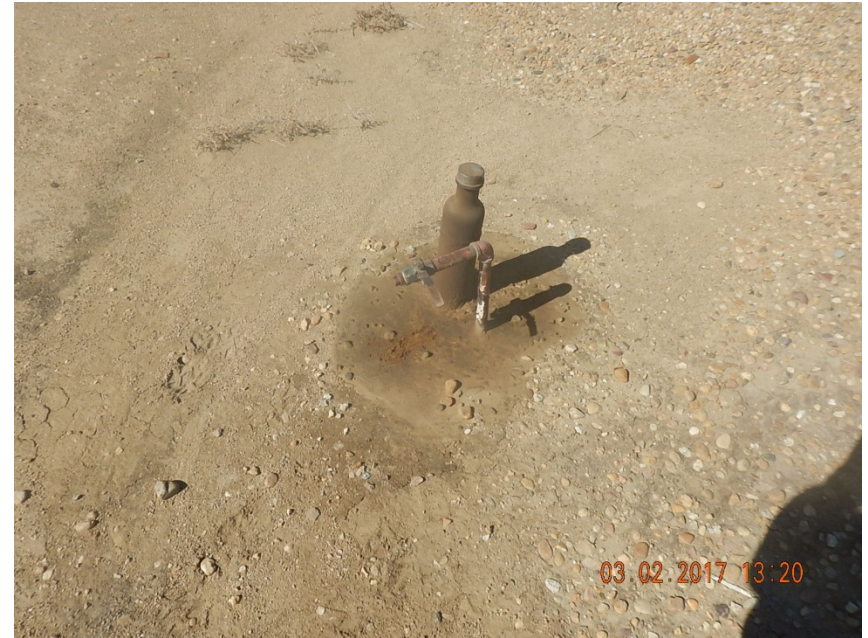
Photo 2: Stained soil at riser
