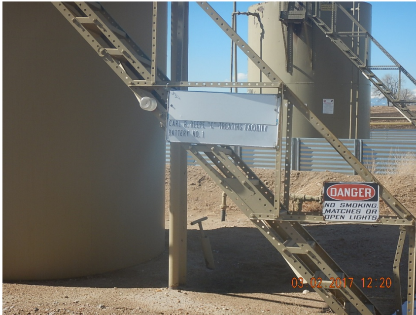
Photo 1: Placard on battery sign is faded, no visible emergency number
