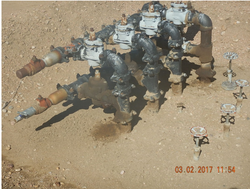
Photo 1: Stained soil at manifold
