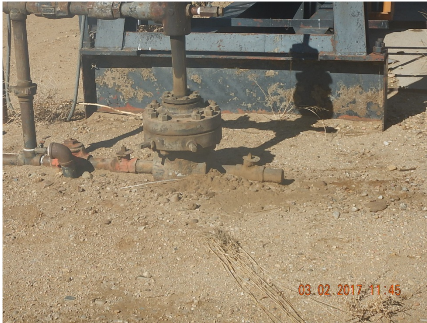
Photo 1: Stained soil at wellhead
