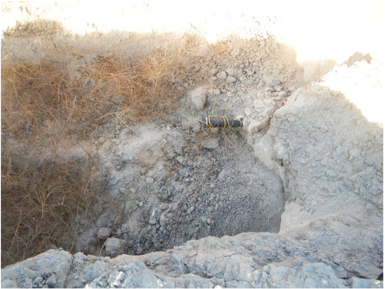
October 14, 2016 view of the northwest end of flowline capped prior to backfilling.
