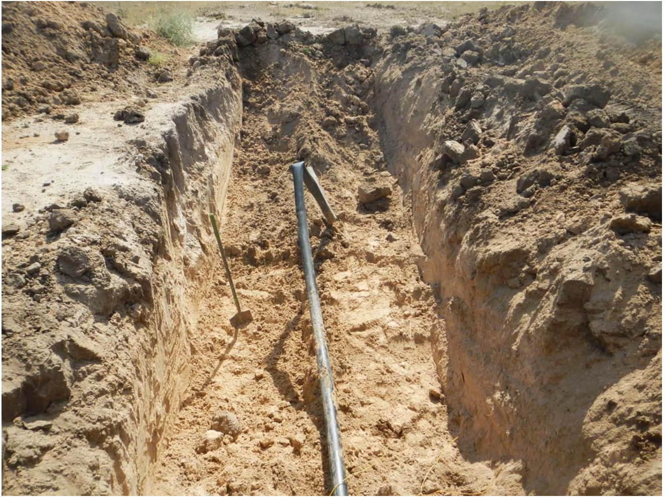
September 21, 2016 view of open excavation prior to cutting out and capping off the damaged flowline segment.
