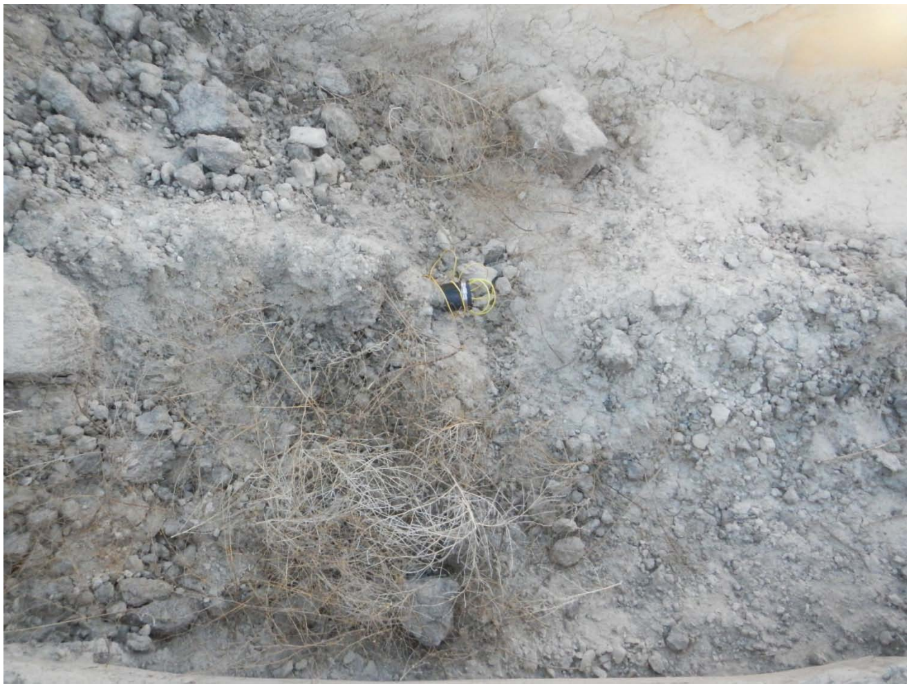
October 14, 2016 view southeast end of flowline capped prior to backfilling.
