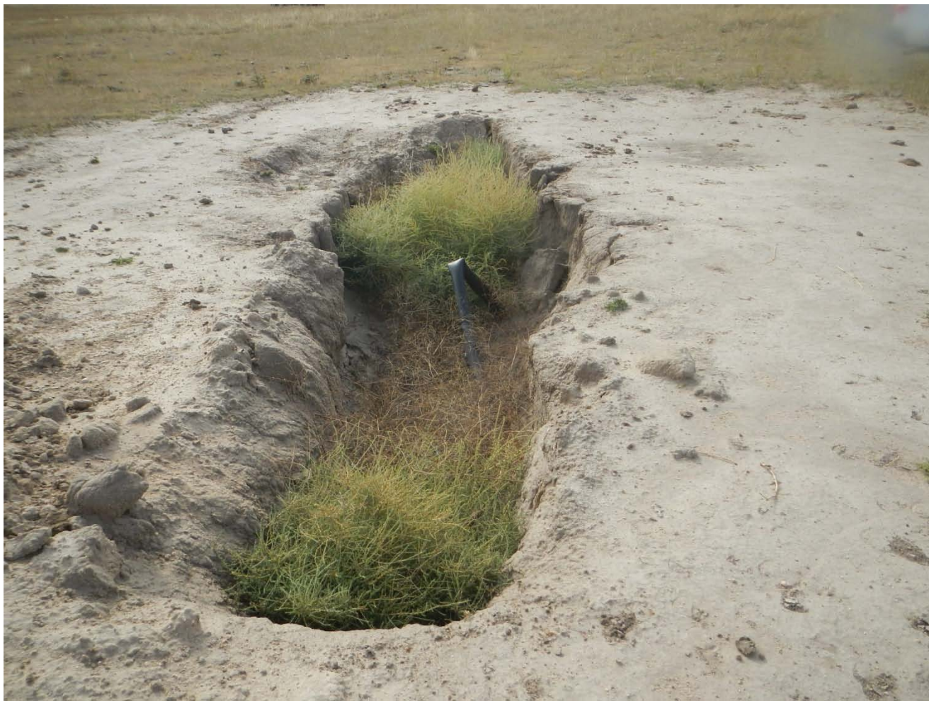
September 21, 2016 view southeast of open flowline leak excavation prior to additional COGCC excavation.
