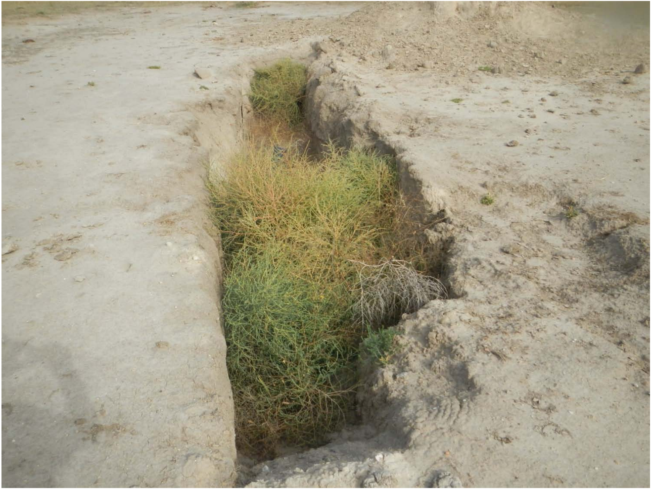
August 15, 2016 view (N) of open flowline leak excavation prior to additional COGCC excavation.
