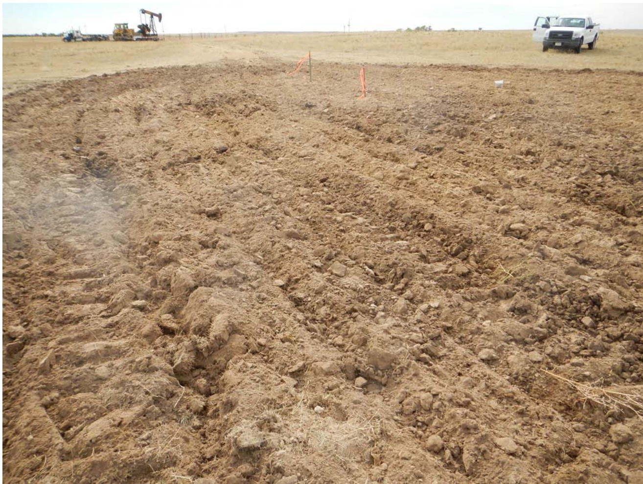
October 14, 2016 view SE across cross ripped area showing flowline cap markers.
