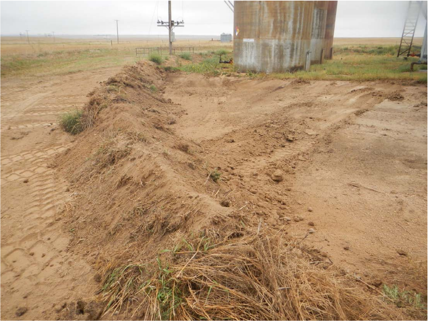
September 22, 2016 view of the rebuilt secondary containment berm.
