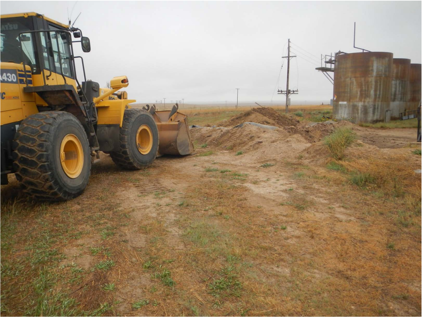
September 22, 2016 view southeast during the removal of impacted soil stockpile from the Spill ID #446079 and Spill ID #447951 spills.
