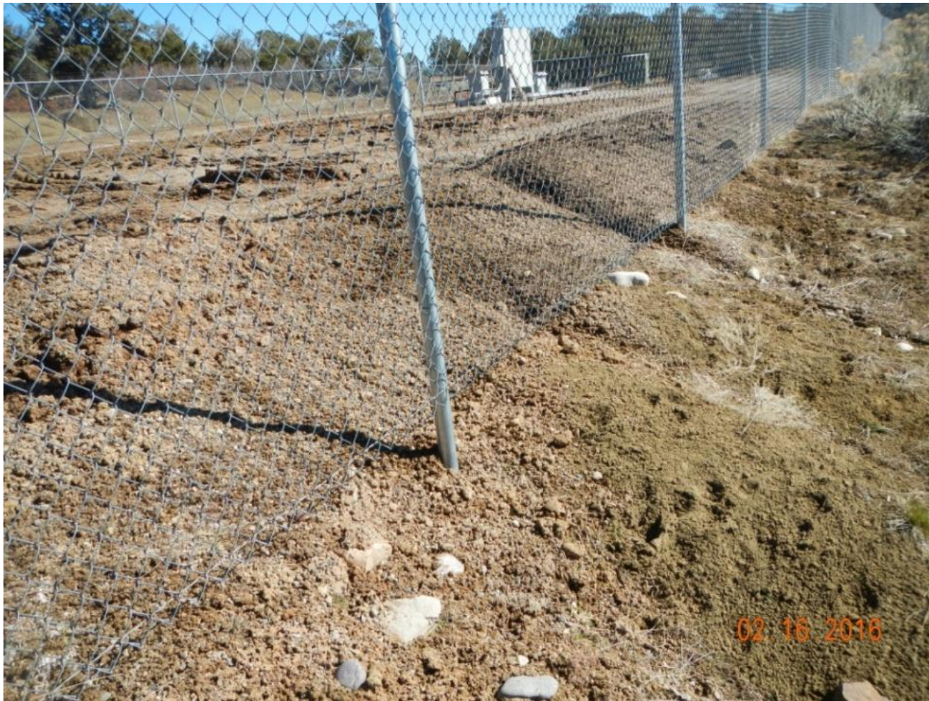
Photo 2: View of erosional channels forming in the southwestern portion of the project area from the southwestern corner facing northeastward.
