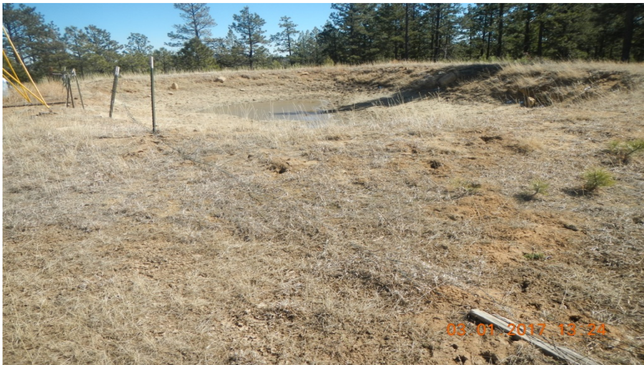
photo 4: The fence around the pit is in disrepair.
