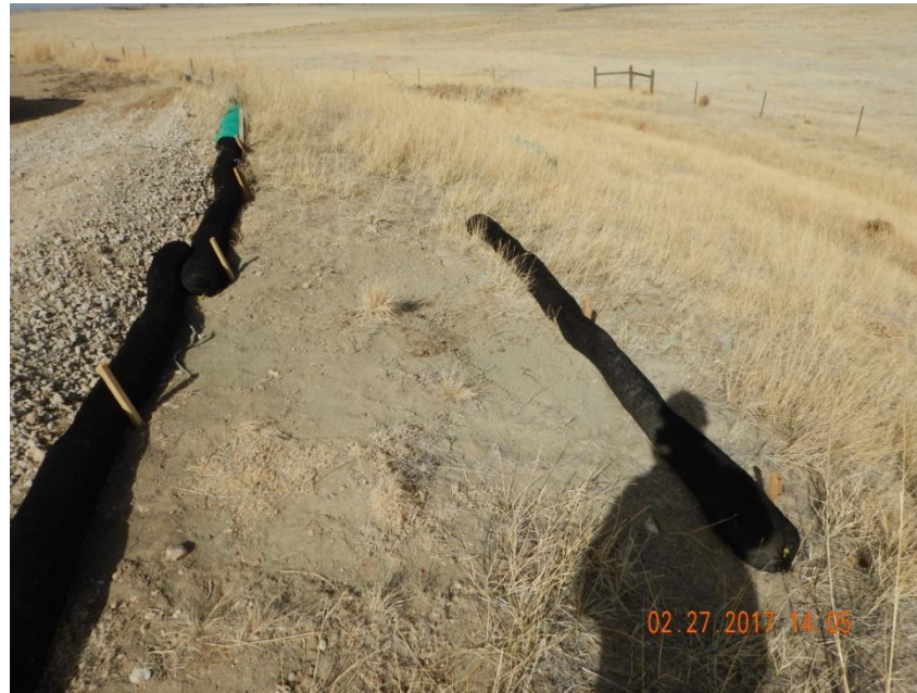
Photo 3. Photo taken from the northeast location along the current interim area, facing North. Gully erosion has been repaired in addition to installing wattles.
