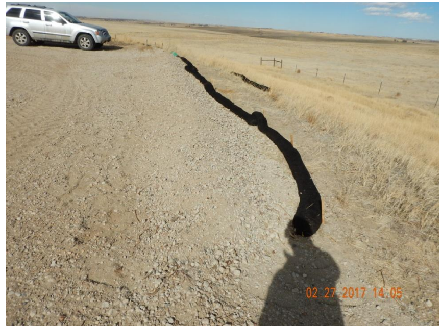
Photo 2. Photo taken from the northeast location, facing North. Wattles have been replaced along the northeast production area and interim areas. Appears gravel has been built up in front of wattle to prevent stormwater runoff from undermining the wattles. Wattles have been overlapped at the joints.
