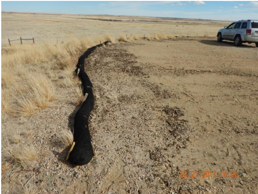
Photo 1. Photo taken from the northeast location, facing East. Wattles have been replaced along the northeast production area and interim areas. Wattles do not appear to be trenched or backfilled along this portion. Stormwater runoff might undermine the wattle and not properly function.
