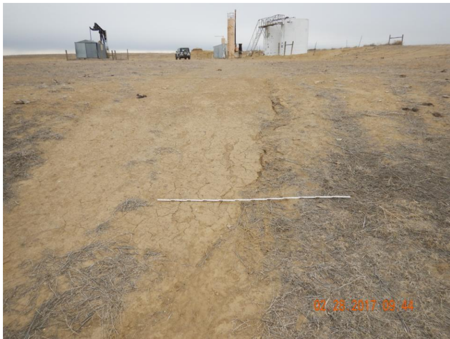
Photo 10: Photo taken from the south end of the location, facing north. Photo shows erosion degradation on the location. Photo shows stormwater and sediment control BMPs have not been installed. 6 foot measuring stick for reference.
