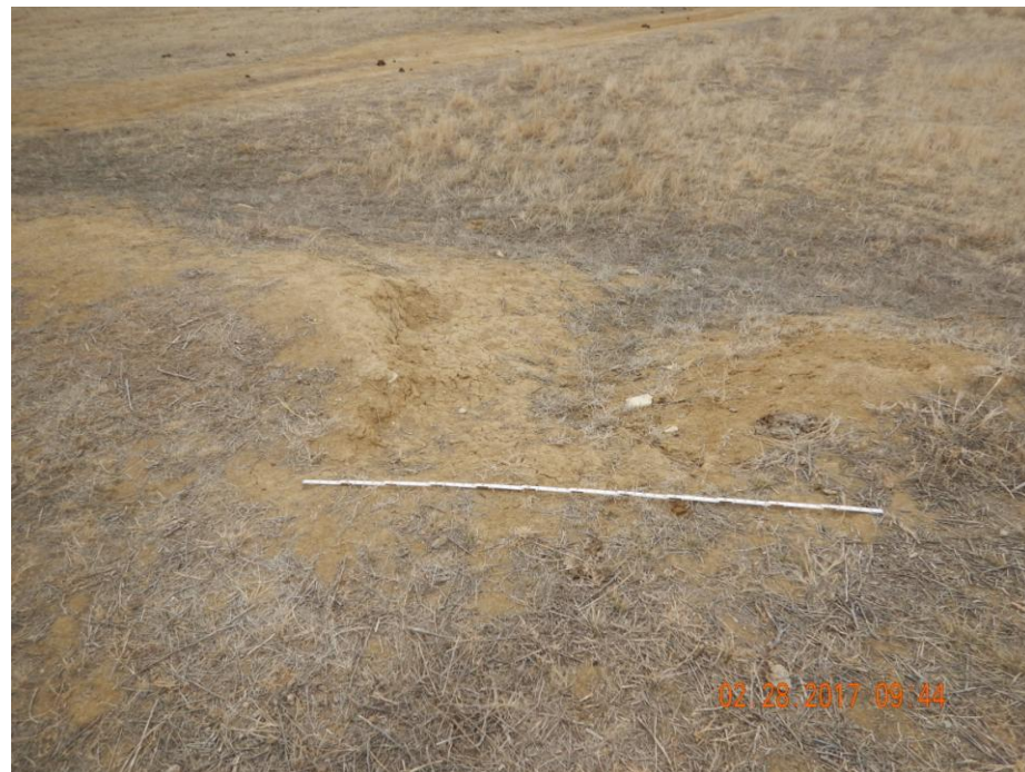
Photo 11: Photo taken from the south end of the location. Photo shows erosion degradation on the location. Photo shows stormwater and sediment control BMPs have not been installed. 6 foot measuring stick for reference.
