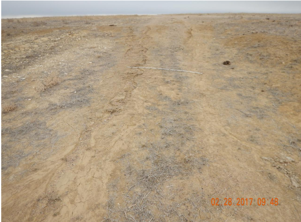
Photo 17: Photo taken from the north end of the location, facing north. Photo shows erosion degradation on the location. Photo shows stormwater and sediment control BMPs have not been installed. 6 foot measuring stick for reference.
