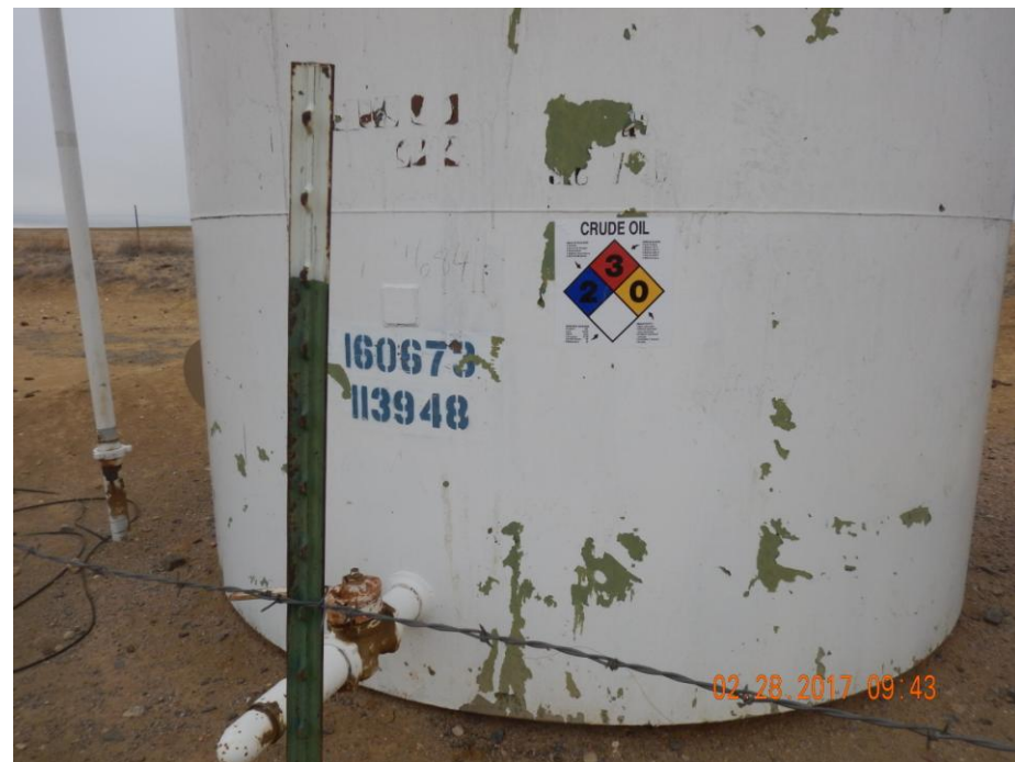
Photo 4: Photo taken from the northern tank, on the southeast end of the location. Photo show placard labels are still missing information such as name of operator, operator's emergency contact telephone number, and tank capacity.
