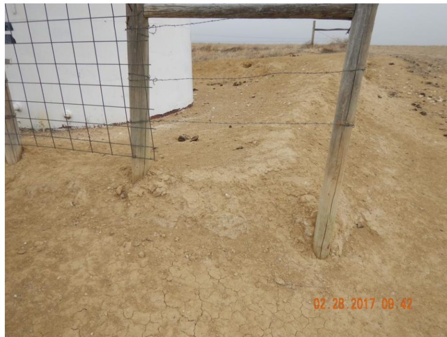
Photo 2: Photo taken southwest corner of the tank battery, on the southeast end of the location facing east. Photo shows berms remain low, insufficient and unrepaired.
