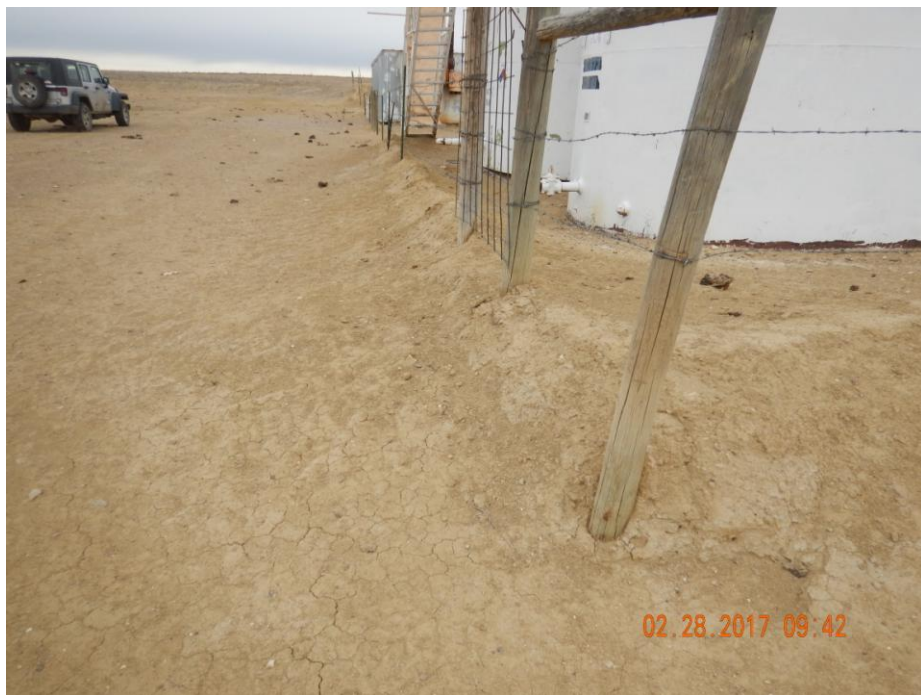
Photo 1: Photo taken southwest corner of the tank battery, on the southeast end of the location facing north. Photo shows berms remain low, insufficient and unrepaired.
