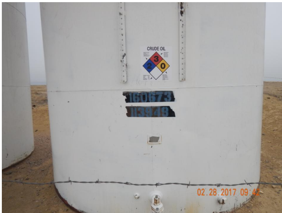
Photo 3: Photo taken from the southern tank, on the southeast end of the location. Photo show placard labels are still missing information such as name of operator, operator's emergency contact telephone number, and tank capacity.
