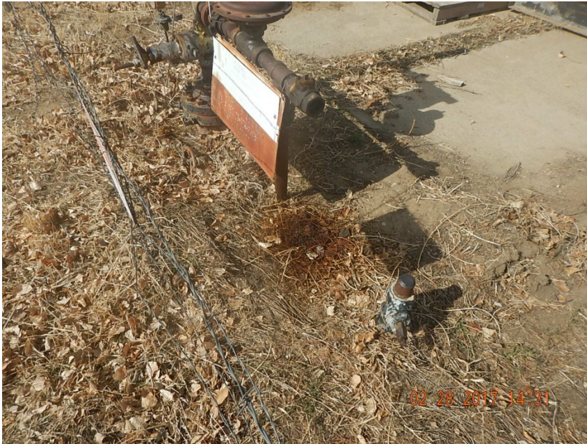
Photo 2: Stained soil at wellhead
