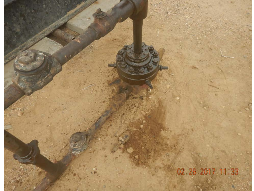
Photo 1: Stained soil at wellhead from prior inspection
