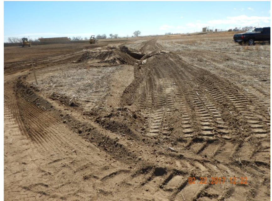
Photo 4. Photo taken from the northwest location, facing South. Ditch and berm BMP installed around perimeter of location.
