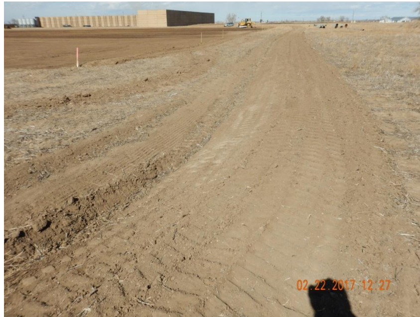
Photo 9. Photo taken from the southeast location, facing North. Ditch and berm BMP installed along perimeter of location.
