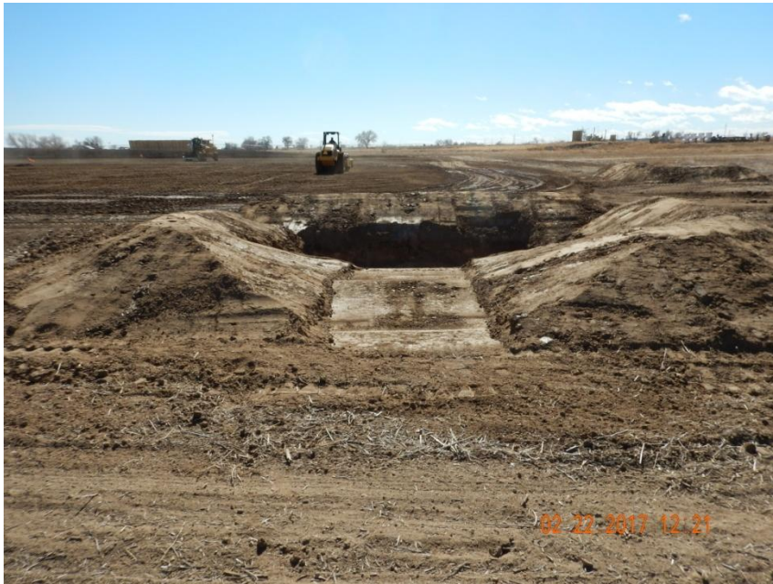
Photo 3. Photo taken from the northwest location, facing South. Sediment trap is IN-PROCESS of being constructed.
