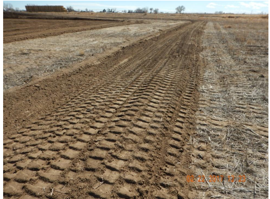
Photo 6. Photo taken from the western location, facing South. Ditch and berm BMP installed around perimeter of location.
