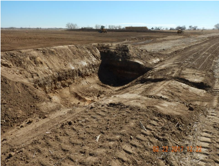
Photo 5. Photo taken from the northwestern location, facing South. Sediment trap is IN-PROCESS of being constructed.
