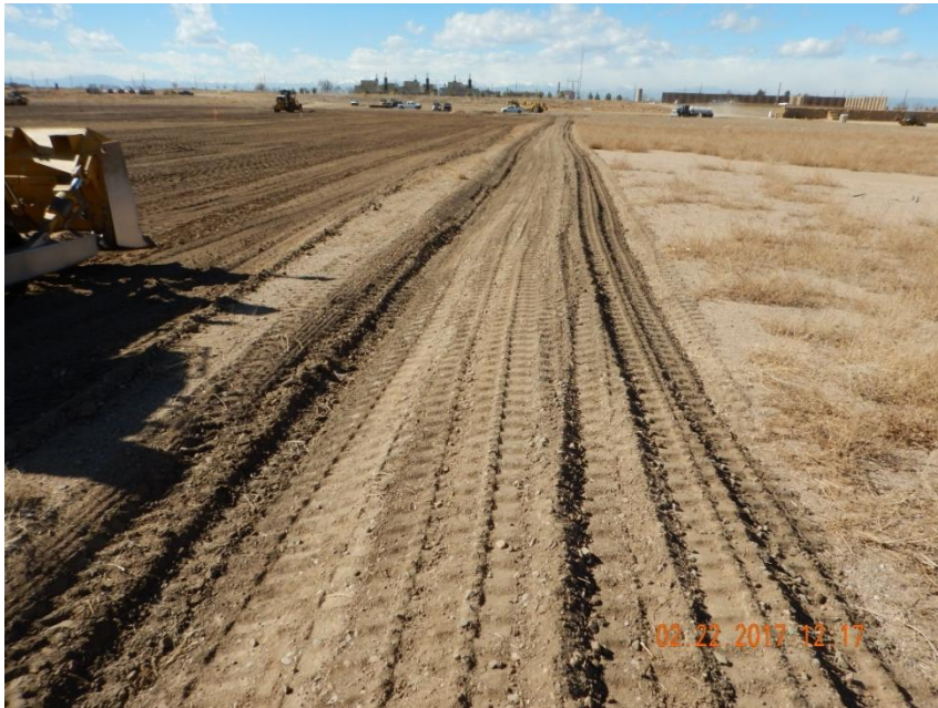
Photo 1. Photo taken from the northern location, facing West. Ditch and berm BMP installed around perimeter of location.
