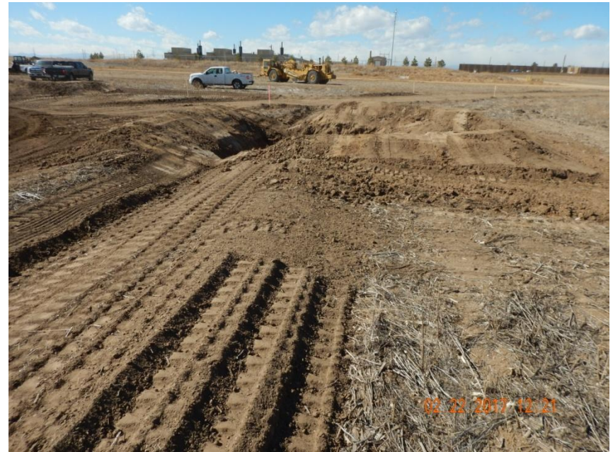
Photo 2. Photo taken from the northwest location, facing West. Sediment trap is IN-PROCESS of being constructed.
