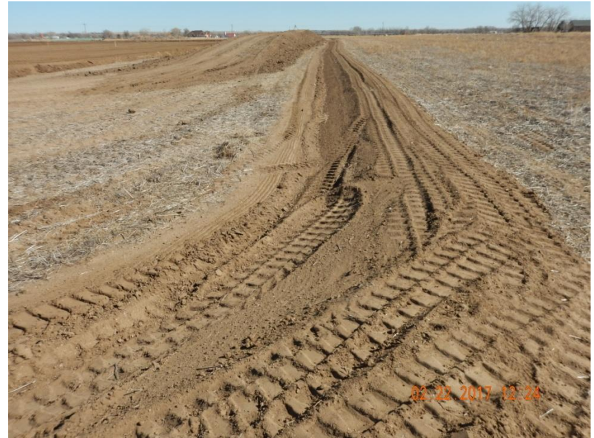
Photo 8. Photo taken from the southwest location, facing East. Ditch and berm BMP installed around perimeter of location.
