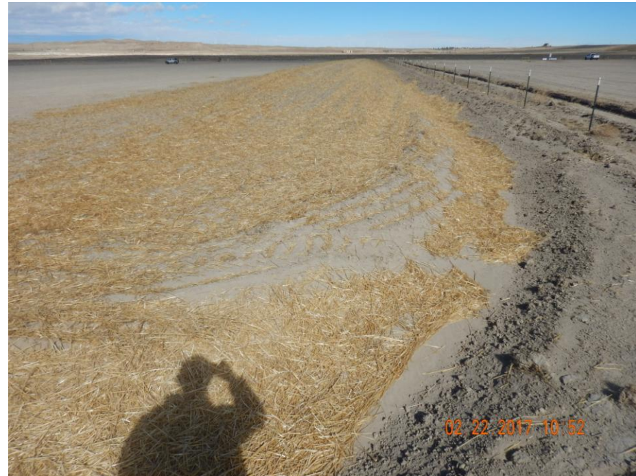
Photo 15: Photo taken from the southeast corner of the location, facing north. Photo shows stormwater control ditch along eastern perimeter of the location. Photo also shows topsoil berm. Topsoil appears to have been seeded and crimped to stabilize soil.
