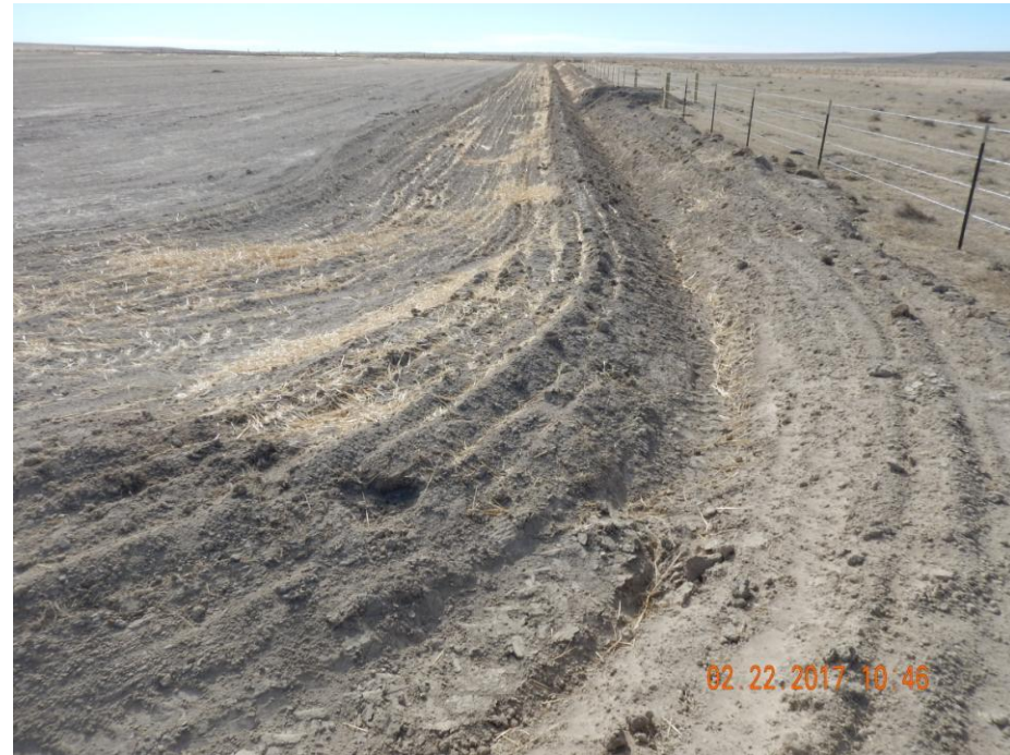
Photo 8: Photo taken from the northwest corner of the location, facing south. Photo shows stormwater and sediment control ditch along northern perimeter of location
