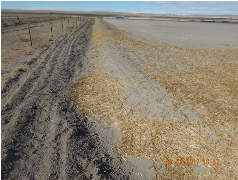
Photo 14: Photo taken from the southeast corner of the location, facing west. Photo shows stormwater control ditch along southern perimeter of the location.
