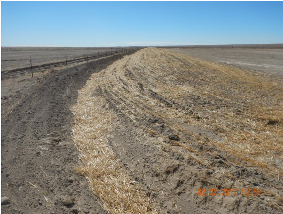
Photo 16: Photo taken from the northeast corner of the location, facing south. Photo shows stormwater control ditch along eastern perimeter of the location. Photo also shows topsoil berm. Topsoil appears to have been seeded and crimped to stabilize soil.
