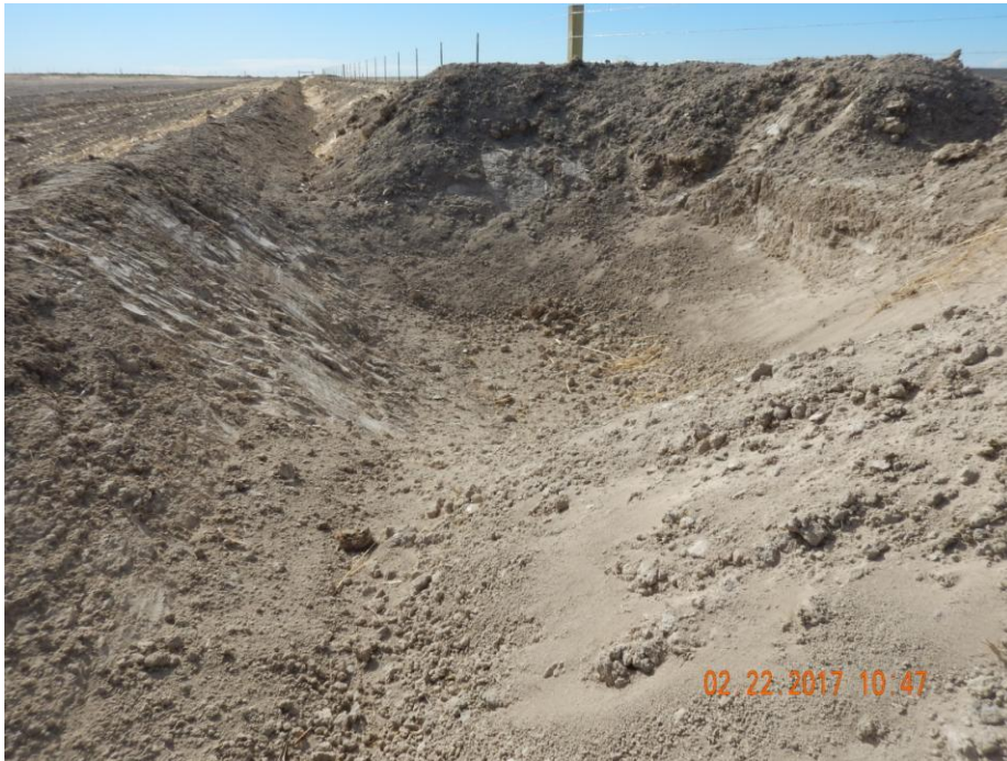
Photo 9: Photo taken from the west end of the location. Photo of sediment trap used as a stormwater and sediment control BMP. Sediment trap does not have sufficient inlet and outlet protection. Also appears that outlet of trap is higher in elevation than the stormwater ditch and the constructed location.
