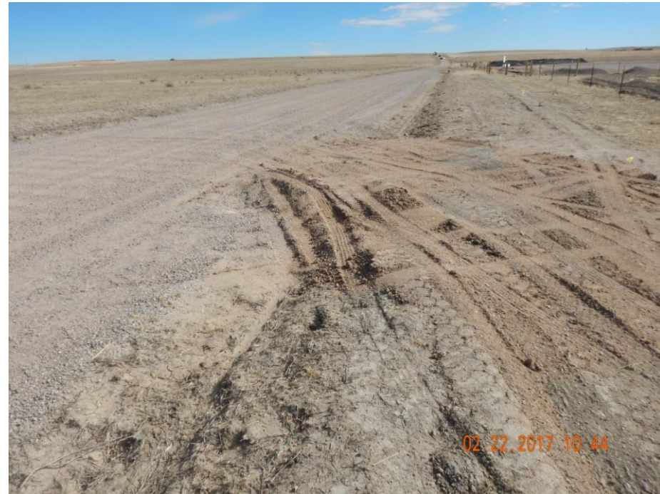
Photo 6: Photo taken from the access road adjacent to the location entrance on the north end of the location. Photo shows stormwater control ditch at access road has been filled with soil, and is no longer in proper functioning conduction.
