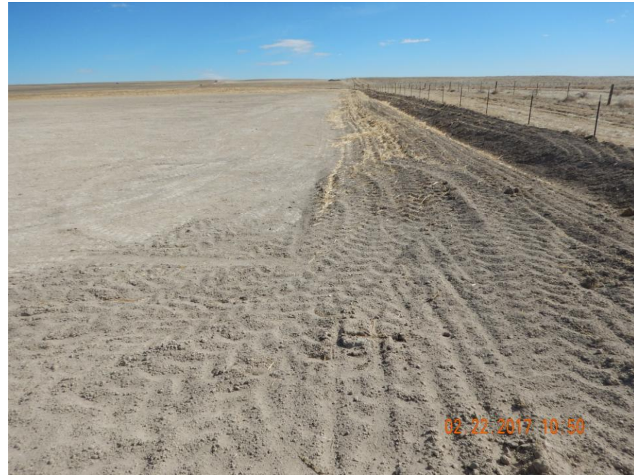
Photo 12: Photo taken from the southwest corner of the location, facing east. Photo shows stormwater control ditch along southern perimeter of the location.
