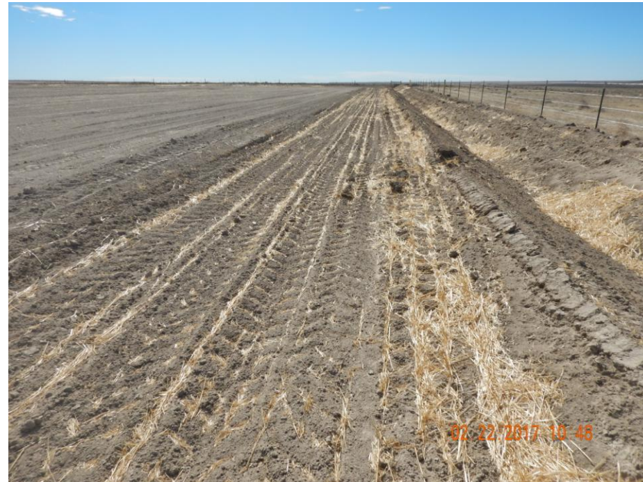
Photo 10: Photo taken from the west end of the location, facing south. Photo shows what appears to be a “spill way” constructed adjacent to the stormwater ditch. “Spill way” appears to have been seeded and stabilized with crimped straw.
