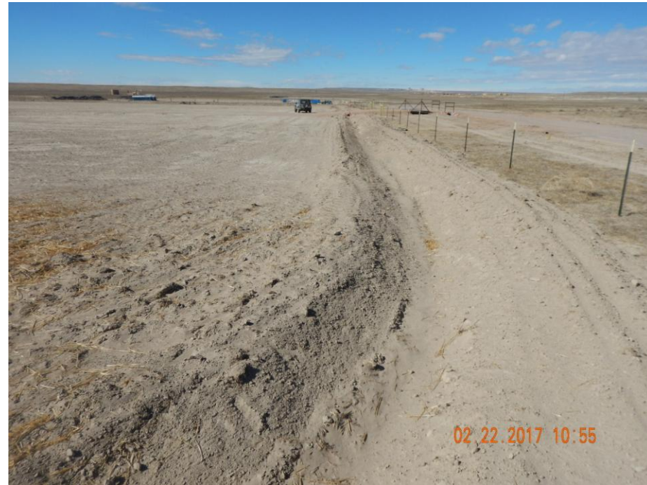
Photo 17: Photo taken from the northeast corner of the location, facing west. Photo shows stormwater control ditch along eastern perimeter of the location.
