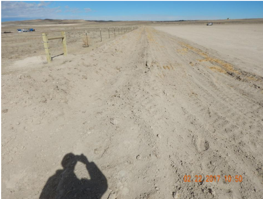
Photo 11: Photo taken from the southwest corner of the location, facing north. Photo shows ditch and “spill way” on west end of location used as stormwater and sediment control BMPs
