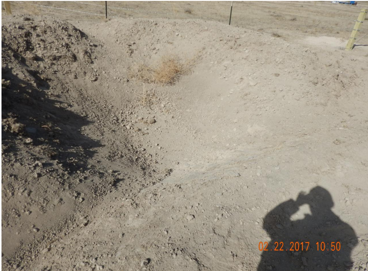
Photo 13: Photo taken from the southwest corner of the location. Photo shows stormwater and sediment control trap. Sediment trap does not have sufficient inlet and outlet protection.
