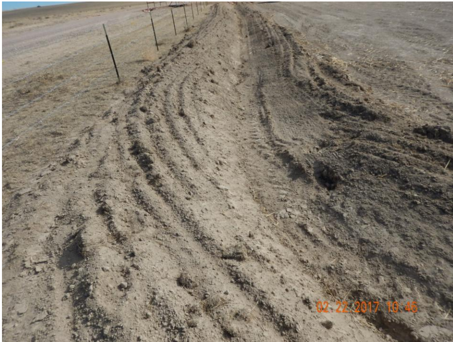
Photo 7: Photo taken from the northwest corner of the location, facing east. Photo shows stormwater and sediment control ditch along northern perimeter of location.
