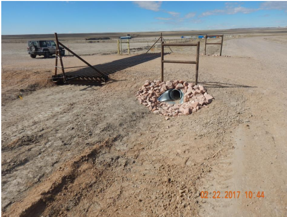
Photo 5: Photo taken from the location entrance on the north end of the location, facing west. Photo shows vehicle tracking BMP (cattle guard) and culvert with armor.
