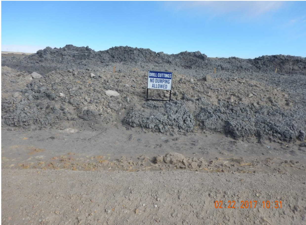
Photo 14: Photo taken from the north end of the location. Photo shows drill cuttings stored on the northeast. A berm has been constructed along the perimeter of the drill cuttings.
