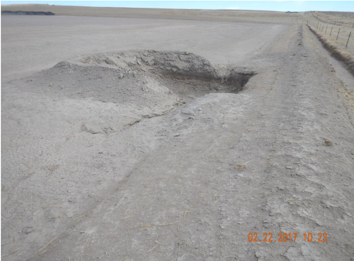
Photo 7: Photo taken from the south end of the location, facing east. Photo of sediment trap. Sediment trap appears inadequate and improperly constructed. Sediment trap has insufficient inlet protection and has gully erosion forming on the location. It is unclear as to why operator constructed BMP in such a manner, as the trap does not have an outlet that would allow water to flow out when it reaches capacity.
