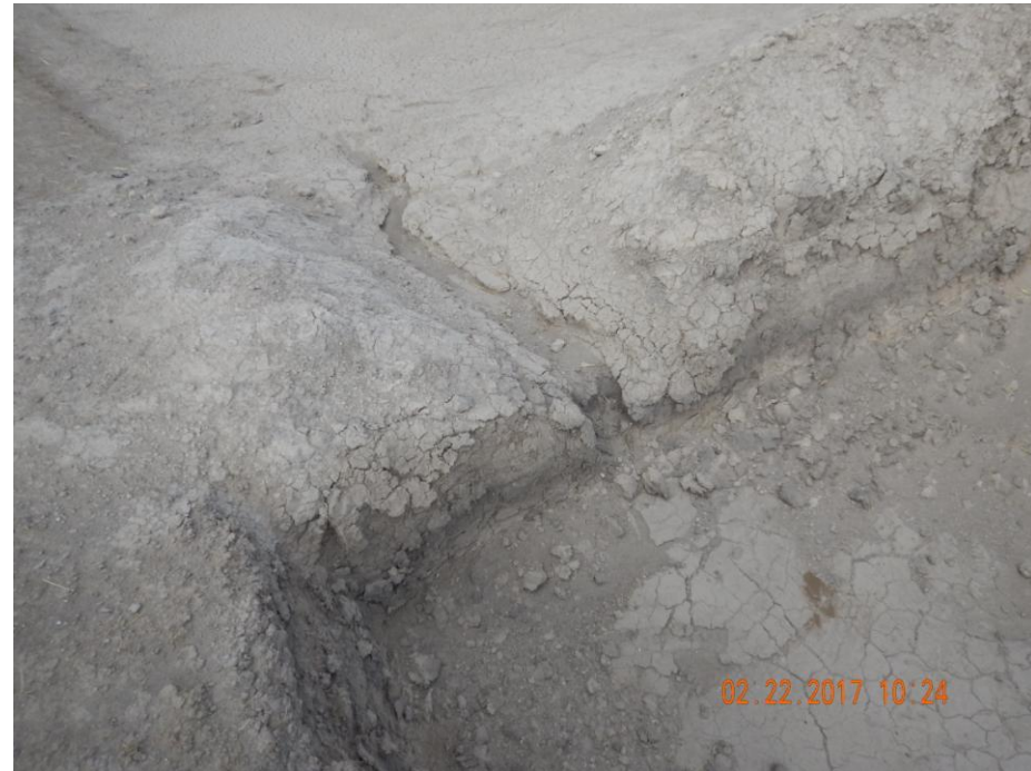
Photo 9: Photo taken from the east end of the location. Photo shows gulley erosion forming at sediment trap due to insufficient inlet protection.
