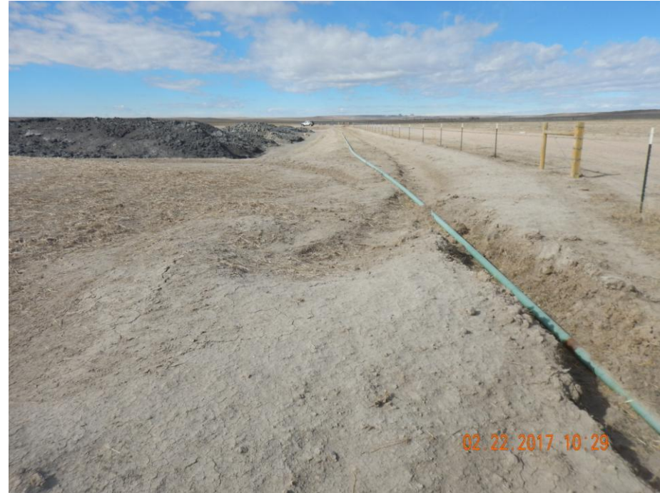
Photo 13: Photo taken from the northeast end of the location, facing south. Photo shows stormwater and sediment control ditch along the northern perimeter of the location.
