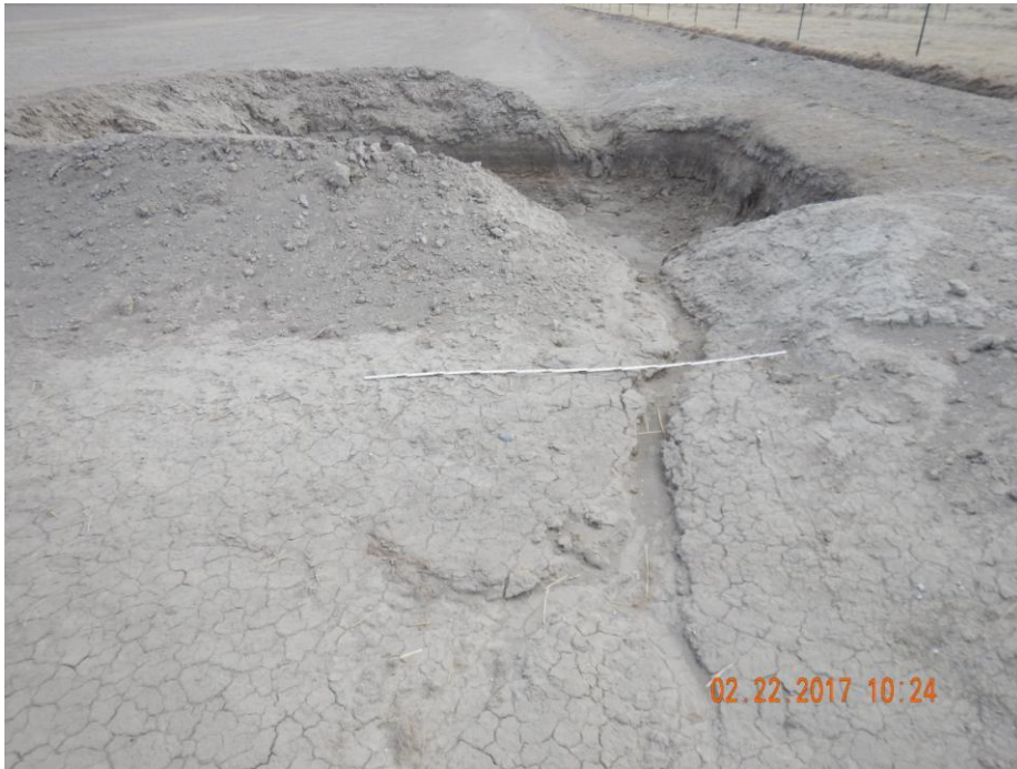
Photo 8: Photo taken from the east end of the location. Photo shows gulley erosion forming at sediment trap due to insufficient inlet protection. 6 foot measuring stick for reference.
