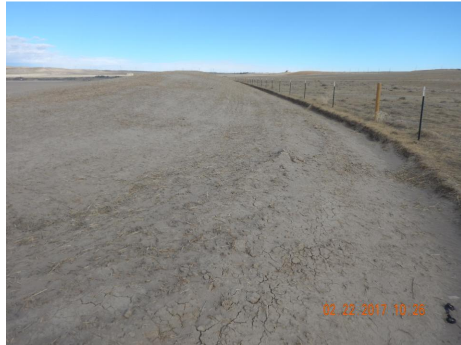
Photo 11: Photo taken from the southeast end of the location, facing north. Photo shows stormwater and sediment control ditch along the eastern perimeter of the location. Photo also shows location of topsoil berm. Topsoil berm appears to have been recently seeded, and crimped to stabilize soil.
