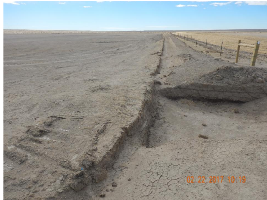
Photo 4: Photo taken from the northwest end of the location, facing south. Photo shows stormwater control ditch along the western perimeter of the location.
