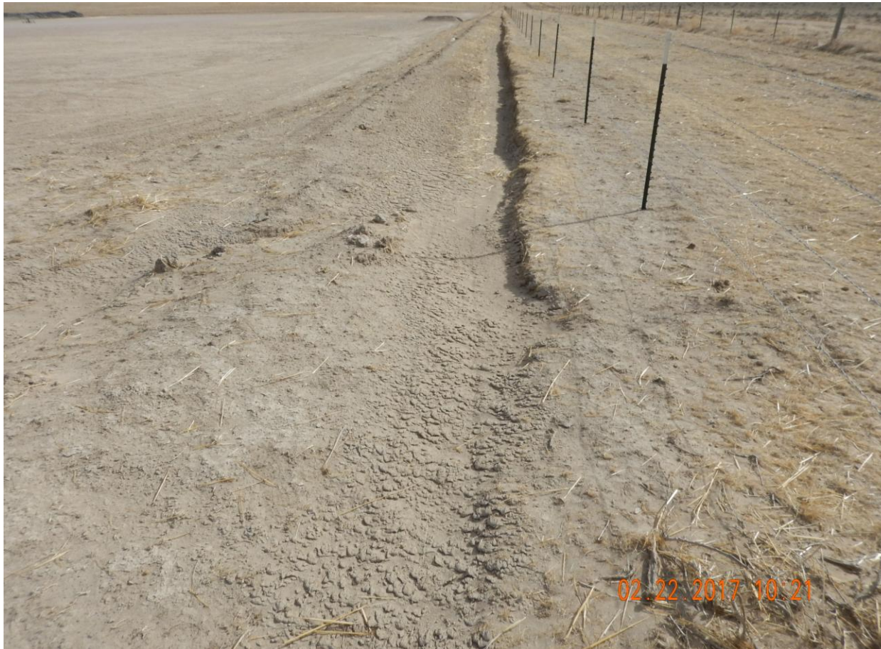
Photo 6: Photo taken from the southwest corner of the location, facing west. Photo shows area of the stormwater ditch along the southern perimeter of the location. Note that leads into the adjacent reference area to the west, and does not have any controls to prevent sediment transport off site, and
