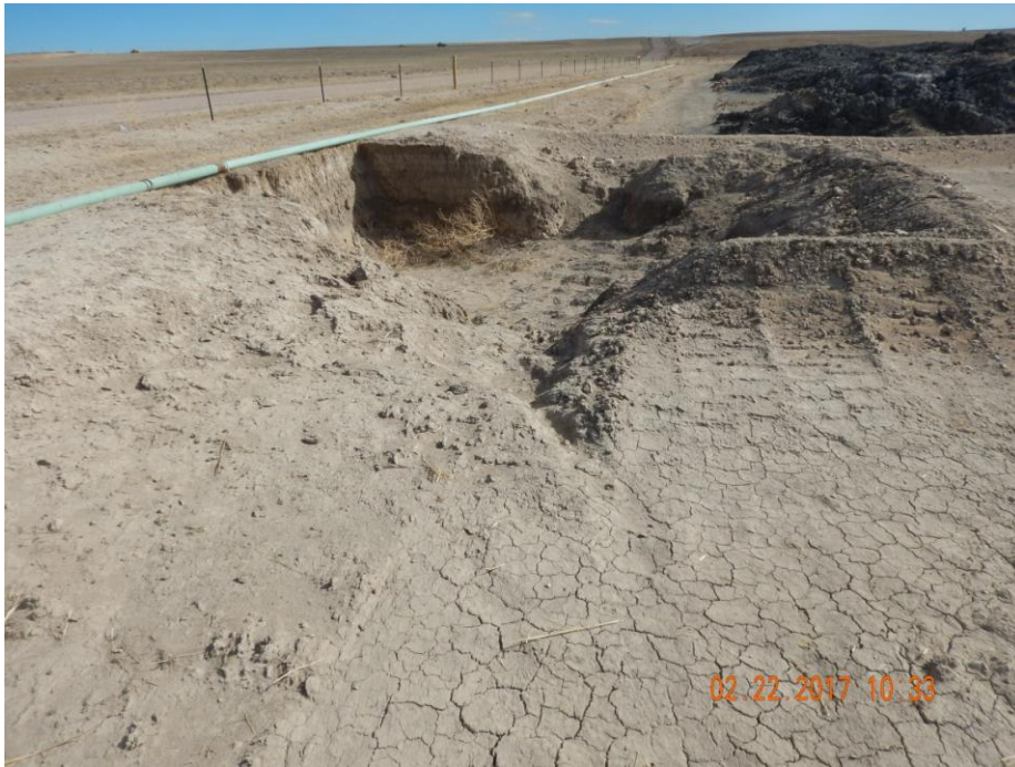
Photo 15: Photo taken from the north end of the location, facing east. Photo of sediment trap. Sediment trap appears inadequate and improperly constructed. Sediment trap has insufficient inlet protection. Due to the way the pad was constructed, it appears stormwater would pool on the north end of the pad as this area is lower in elevation than the adjacent stormwater ditch on the north end of the location.
