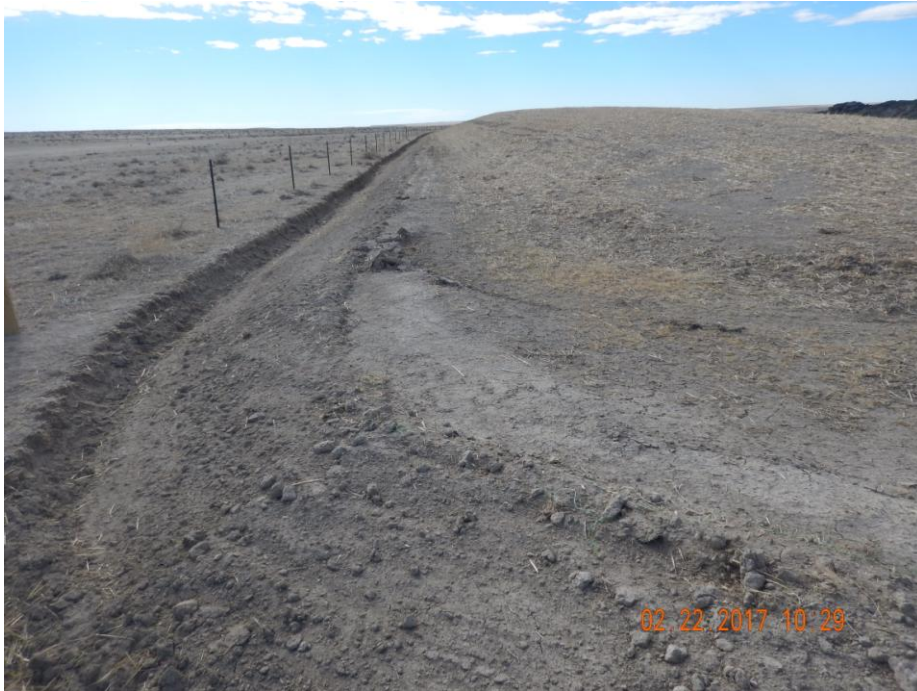
Photo 12: Photo taken from the northeast end of the location, facing south. Photo shows stormwater and sediment control ditch along the eastern perimeter of the location. Photo also shows location of topsoil berm. Topsoil berm appears to have been recently seeded, and crimped to stabilize soil.
