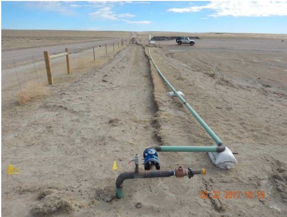
Photo 3: Photo taken from the northwest end of the location, facing east. Photo shows stormwater control ditch along perimeter of the location. Ditch does not appear to properly function.
