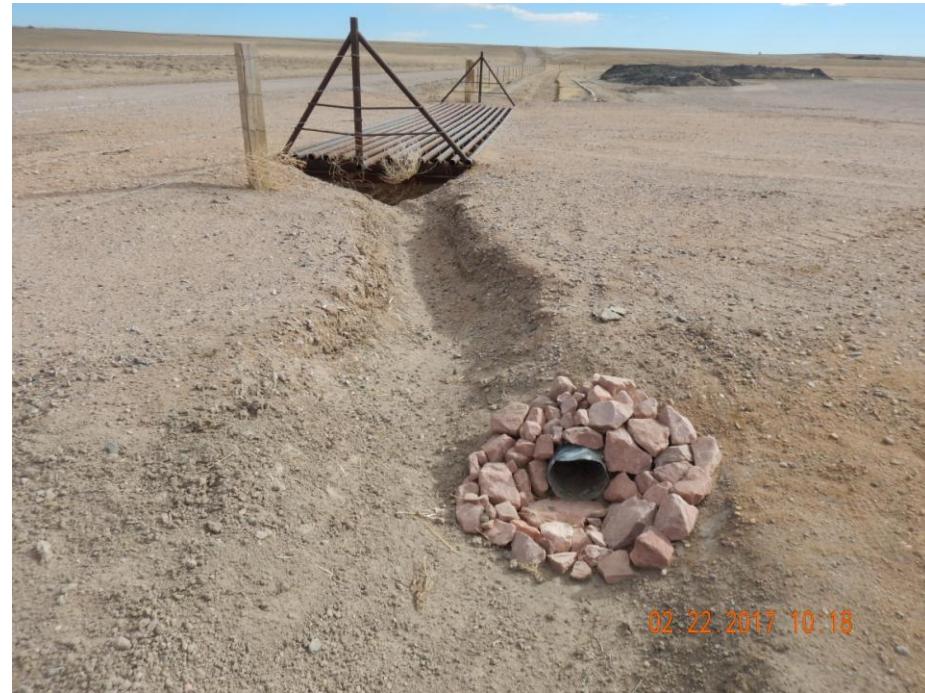
Photo 2: Photo taken from the north end of the location, facing east. Photo shows vehicle tracking BMP at entrance to location and culvert with rock armoring.
