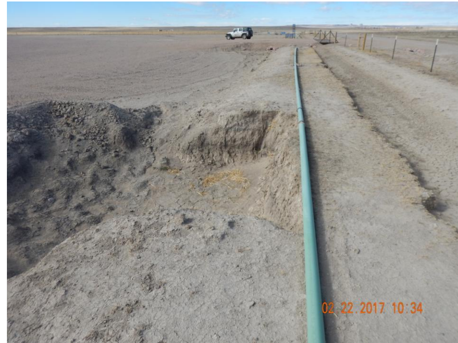
Photo 16: Photo taken from the north end of the location, facing west. Photo of sediment trap. Sediment trap appears inadequate and improperly constructed. Sediment trap has insufficient inlet protection. Due to the way the pad was constructed, it appears stormwater would pool on the north end of the pad, as this area is lower in elevation than the adjacent stormwater ditch on the north end of the location.
