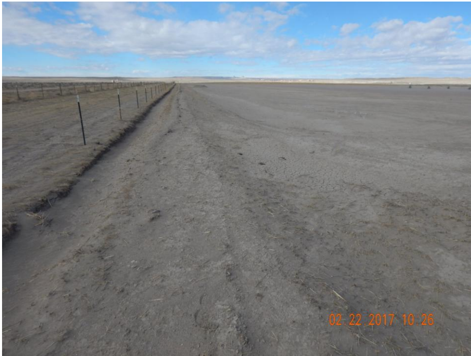
Photo 10: Photo taken from the southeast end of the location, facing west. Photo shows stormwater and sediment control ditch along the southern perimeter of the location.
