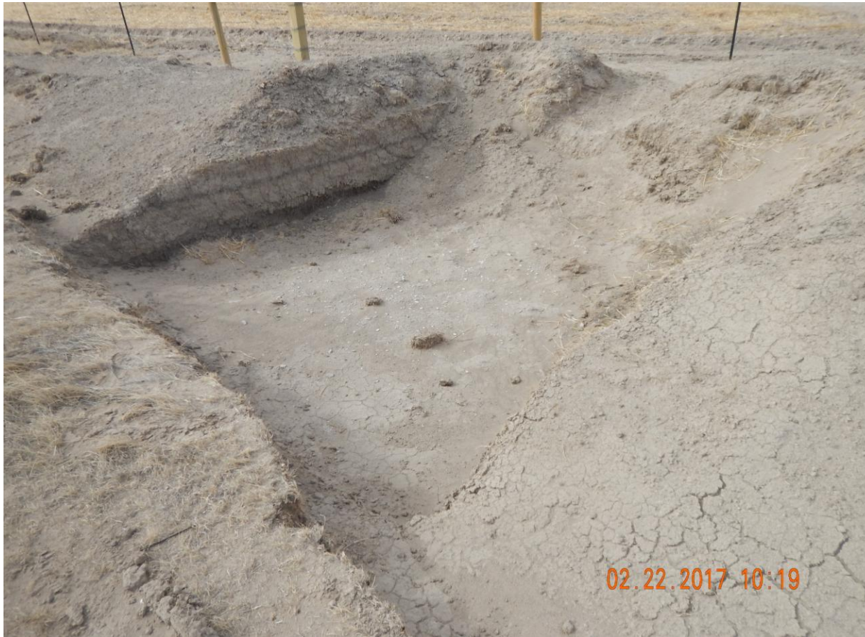
Photo 5: Photo taken from the northwest end of the location. Photo shows sediment trap used as a stormwater and sediment control BMP. Sediment trap appears inadequate and improperly constructed. Sediment trap has insufficient inlet and outlet protection.
