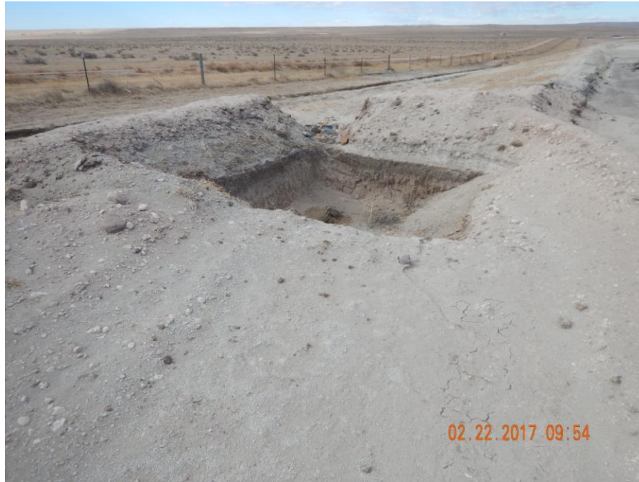
Photo 8: Photo taken from the south end of the location. Photo shows sediment trap used as a stormwater and sediment control BMP. Sediment trap has insufficient inlet protection. Sediment has begun to fill with sediment and will require maintenance.
