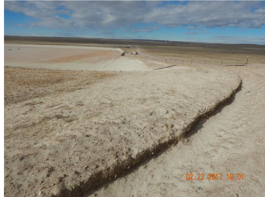
Photo 23: Photo taken from the northeast corner of the location, facing west. Photo shows stormwater control ditch along perimeter of the location.
