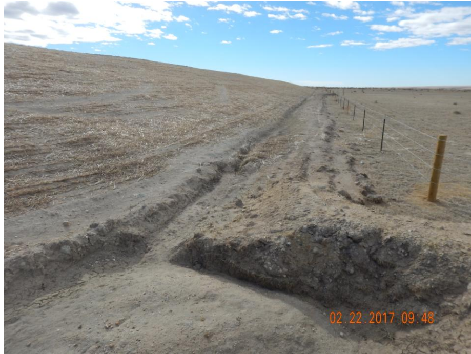
Photo 14: Photo taken from the northwest corner of the location, facing south. Photo shows stormwater control ditch along perimeter of the location. Photo also shows slopes on the west end of the location appear to be seeded, and crimped with straw to stabilize the soil.
