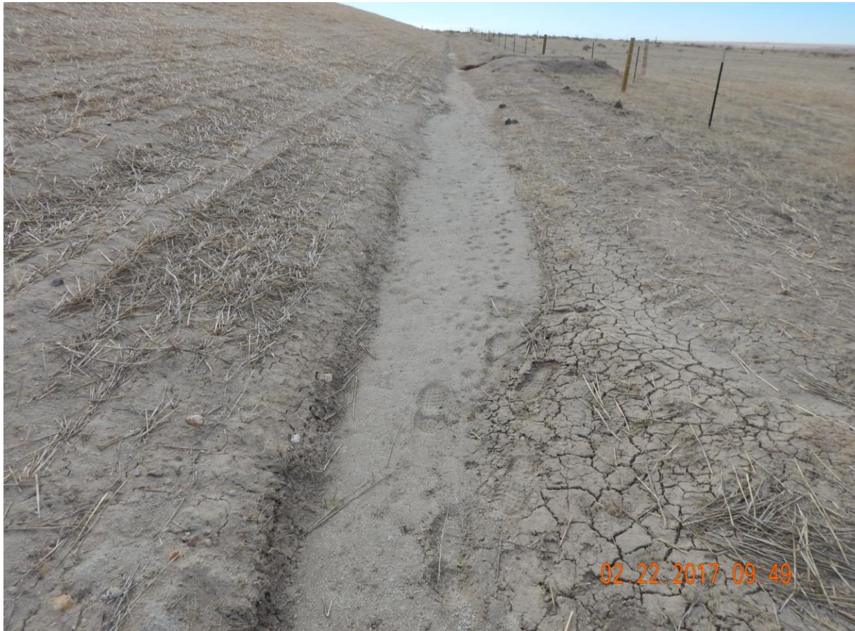
Photo 16: Photo taken from the west end of the location, facing south. Photo shows stormwater ditch has filled with sediment and no longer in proper functioning condition. Ditch will require maintenance.
