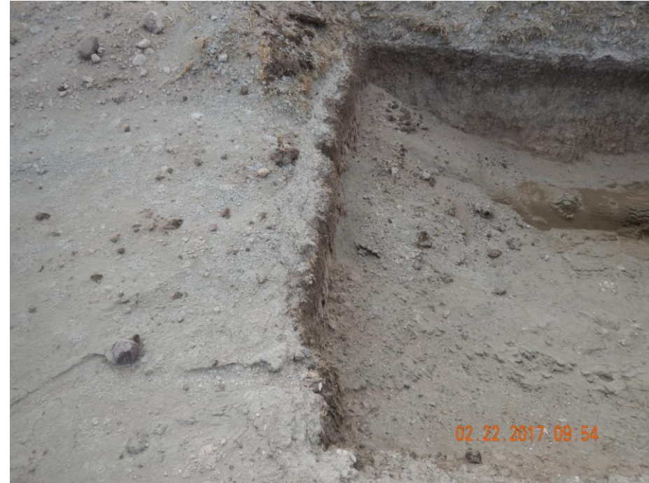
Photo 9: Photo taken from the south end of the location. Photo shows sediment trap used as a stormwater and sediment control BMP. Sediment trap has insufficient inlet protection. Photo shows inlet as been inadequately constructed; it is advised that inlets are constructed with a 2:1 slope, or flatter.
