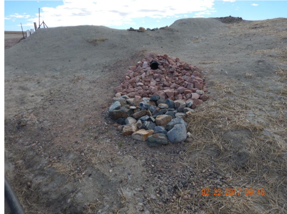
Photo 4: Photo taken from the north end of the location. Photo shows sediment trap used as a stormwater and sediment control BMP. Photo shows armoring around outlet drain, that leads into a stormwater ditch on the north perimeter.
