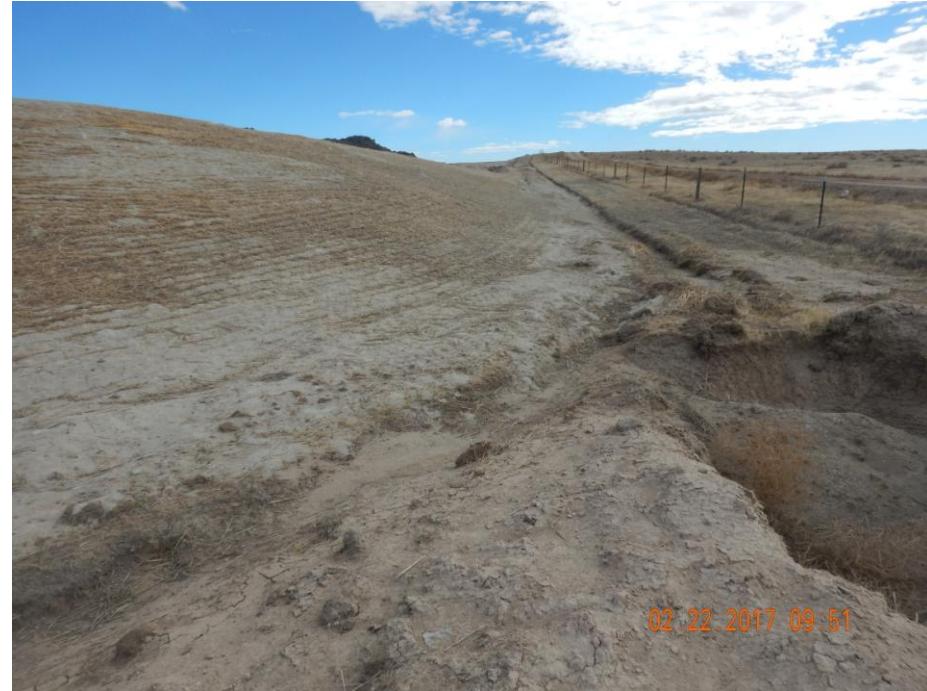
Photo 18: Photo taken from the northwest corner of the location, facing east. Photo shows stormwater control ditch along perimeter of the location. Photo also shows slopes on the south end of the location appear to have been seeded, and crimped with straw to stabilize the soil.
