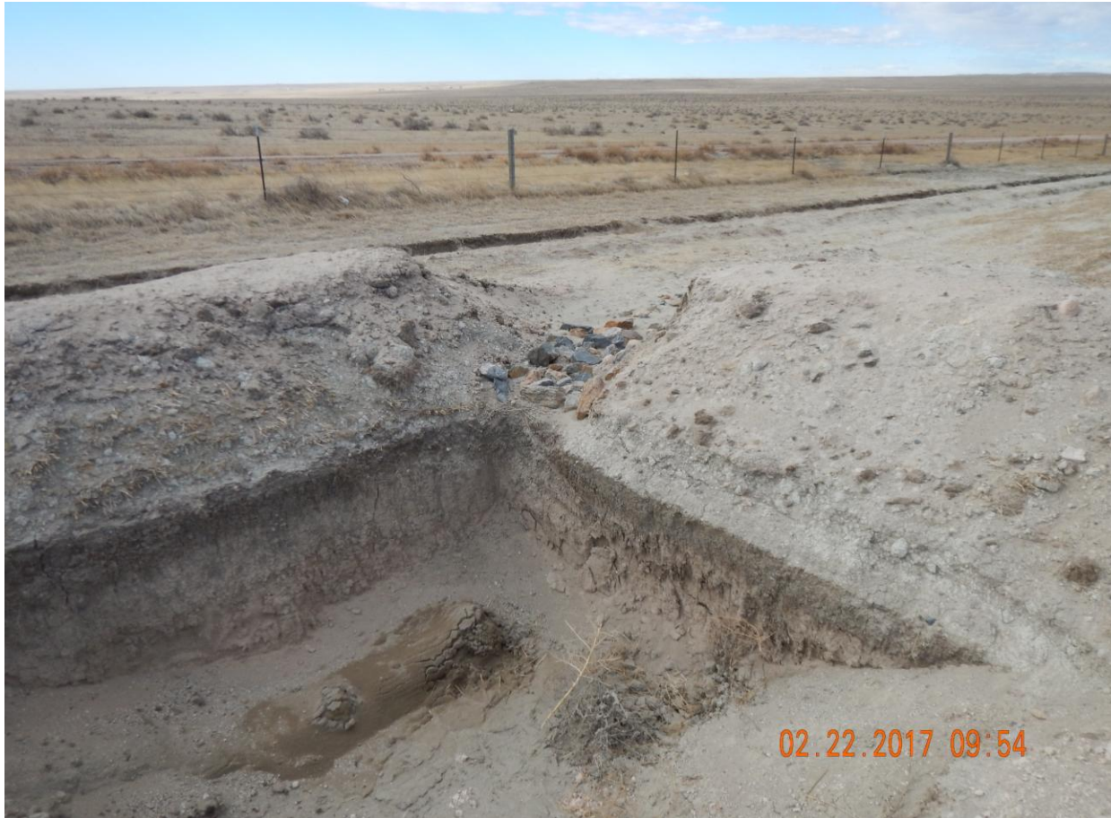
Photo 10: Photo taken from the south end of the location, facing south. Photo shows sediment trap used as a stormwater and sediment control BMP. Photo shows armoring around outlet. Current rock armoring may be insufficient and appears to have filled with sediment.
