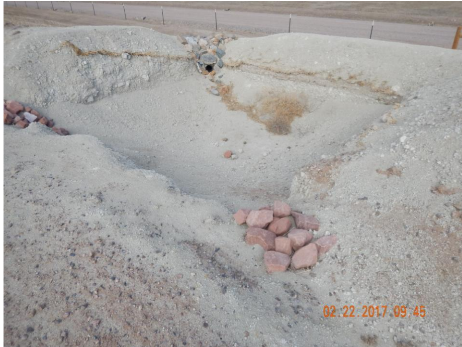
Photo 3: Photo taken from the north end of the location. Photo shows sediment trap used as a stormwater and sediment control BMP. Inlets and outlet contain armoring. Drain incorporated in outlet.
