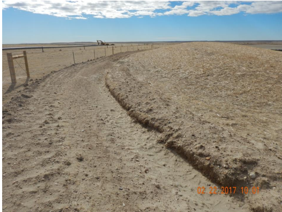
Photo 22: Photo taken from the northeast corner of the location, facing south. Photo shows stormwater control ditch along perimeter of the location. Photo also shows topsoil berm located on the east end of the location. Berm appears to have been seeded, and crimped with straw to stabilize the soil.
