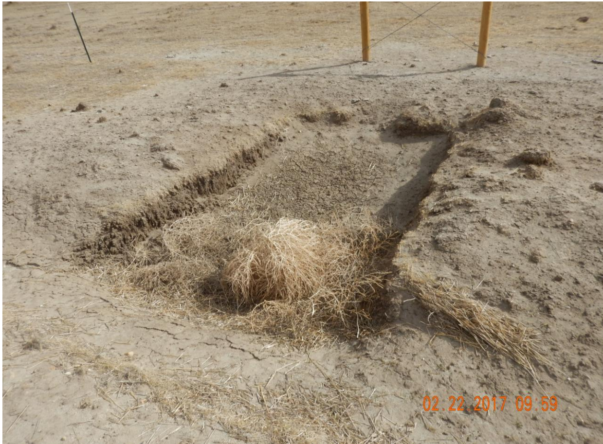
Photo 11: Photo taken from the east end of the location. Photo shows sediment trap used as a stormwater and sediment control BMP. Sediment trap appears inadequate and improperly constructed. Sediment trap has insufficient inlet and outlet protection. Sediment trap appears inadequate and improperly constructed.
