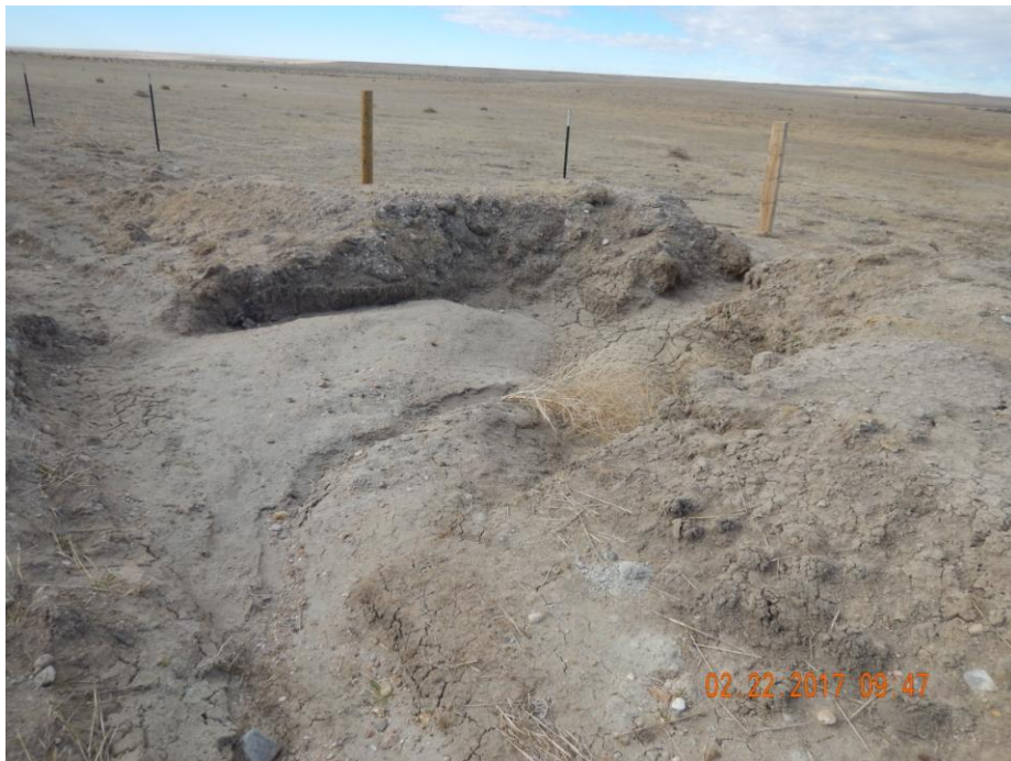
Photo 5: Photo taken from the northwest end of the location. Photo shows sediment trap used as a stormwater and sediment control BMP. Sediment trap appears inadequate and improperly constructed. Sediment trap has insufficient inlet and outlet protection. Photo shows trap has filled with sediment and will require maintenance.
