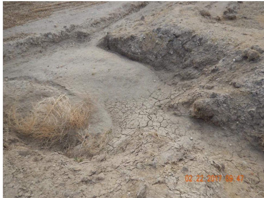
Photo 6: Photo taken from the northwest end of the location. Photo shows sediment trap used as a stormwater and sediment control BMP. Sediment trap appears inadequate and improperly constructed. Sediment trap has insufficient inlet and outlet protection. Photo shows trap has filled with sediment and will require maintenance.
