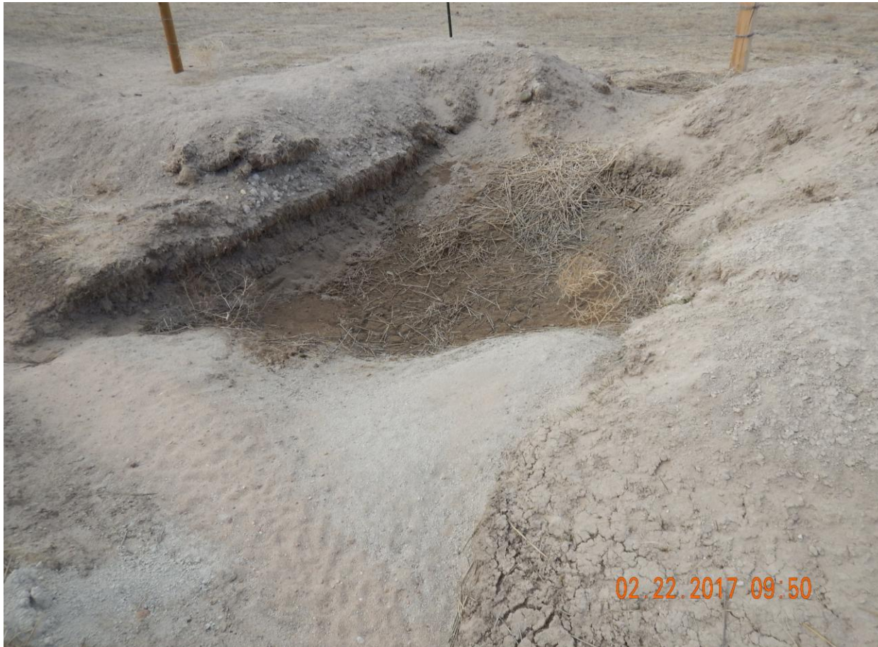
Photo 7: Photo taken from the west end of the location. Photo shows sediment trap used as a stormwater and sediment control BMP. Sediment trap appears inadequate and improperly constructed. Sediment trap has insufficient inlet and outlet protection. Photo shows trap has filled with sediment and will require maintenance.
