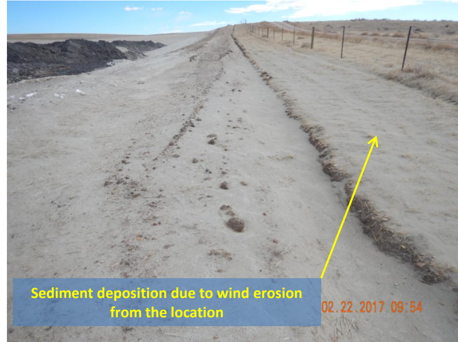
Photo 20: Photo taken from the south end of the location, facing east. Photo shows stormwater ditch has filled with sediment and no longer in proper functioning condition. Ditch will require maintenance. Photo also shows areas outside of the location where wind erosion has deposited sediment from the location.
