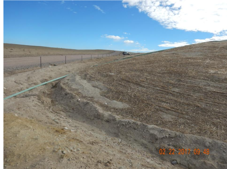
Photo 15: Photo taken from the northwest corner of the location, facing east. Photo shows stormwater control ditch along perimeter of the location.
