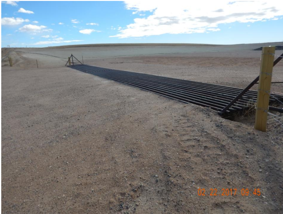
Photo 1: Photo taken from the north end of the location, facing southeast. Photo shows vehicle tracking BMP as entrance to location.
