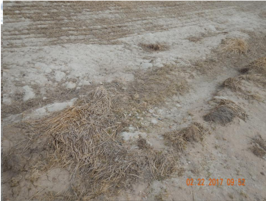
Photo 19: Photo taken from the south end of the location. Photo shows stormwater ditch has filled with sediment and no longer in proper functioning condition. Ditch will require maintenance.
