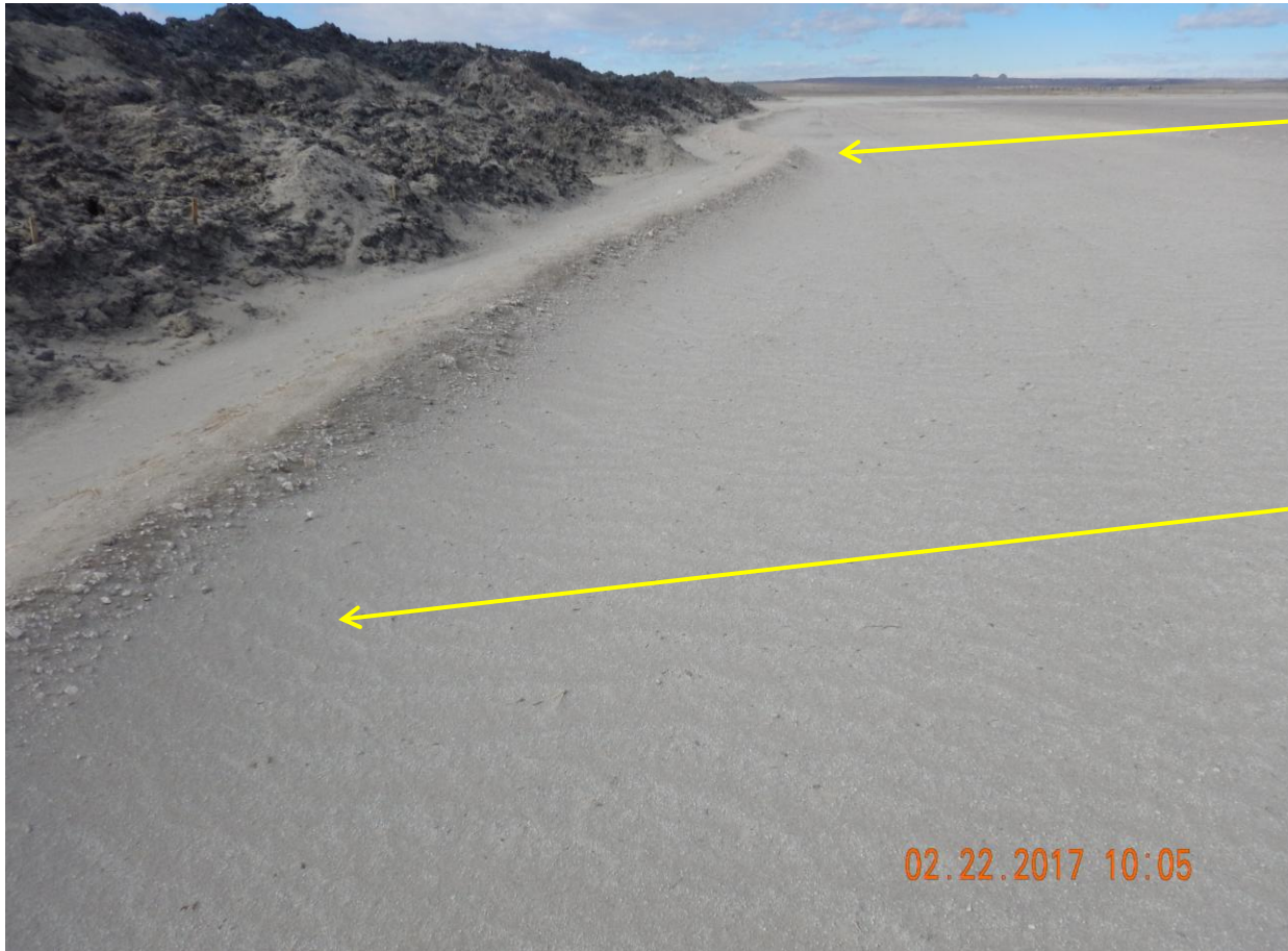
Photo 24: Photo taken from the south end of the location, facing west. Photo shows berm constructed around drill cuttings. Photo also shows sediment deposition due to wind erosion occurring on and from the location.
