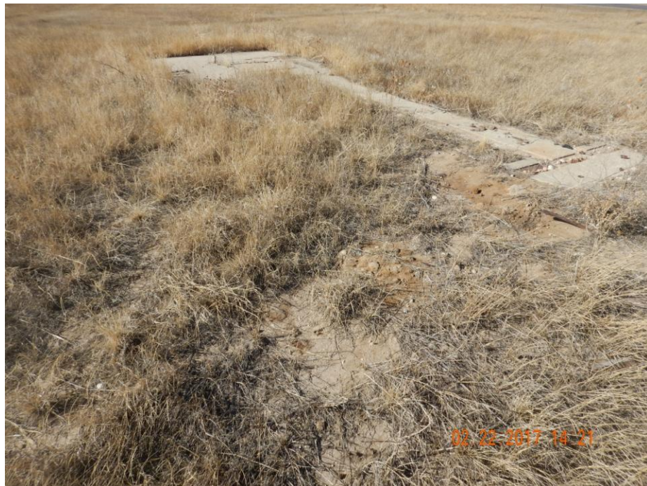
Photo 3: Photo shows concrete pad remaining at well.
