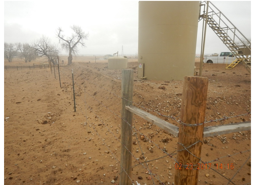
Photo 1: Berms and fence repaired
