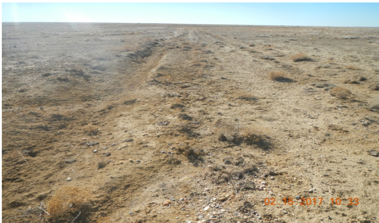
photo 1: Facing south along the access road. There are signs of erosion along the road.
