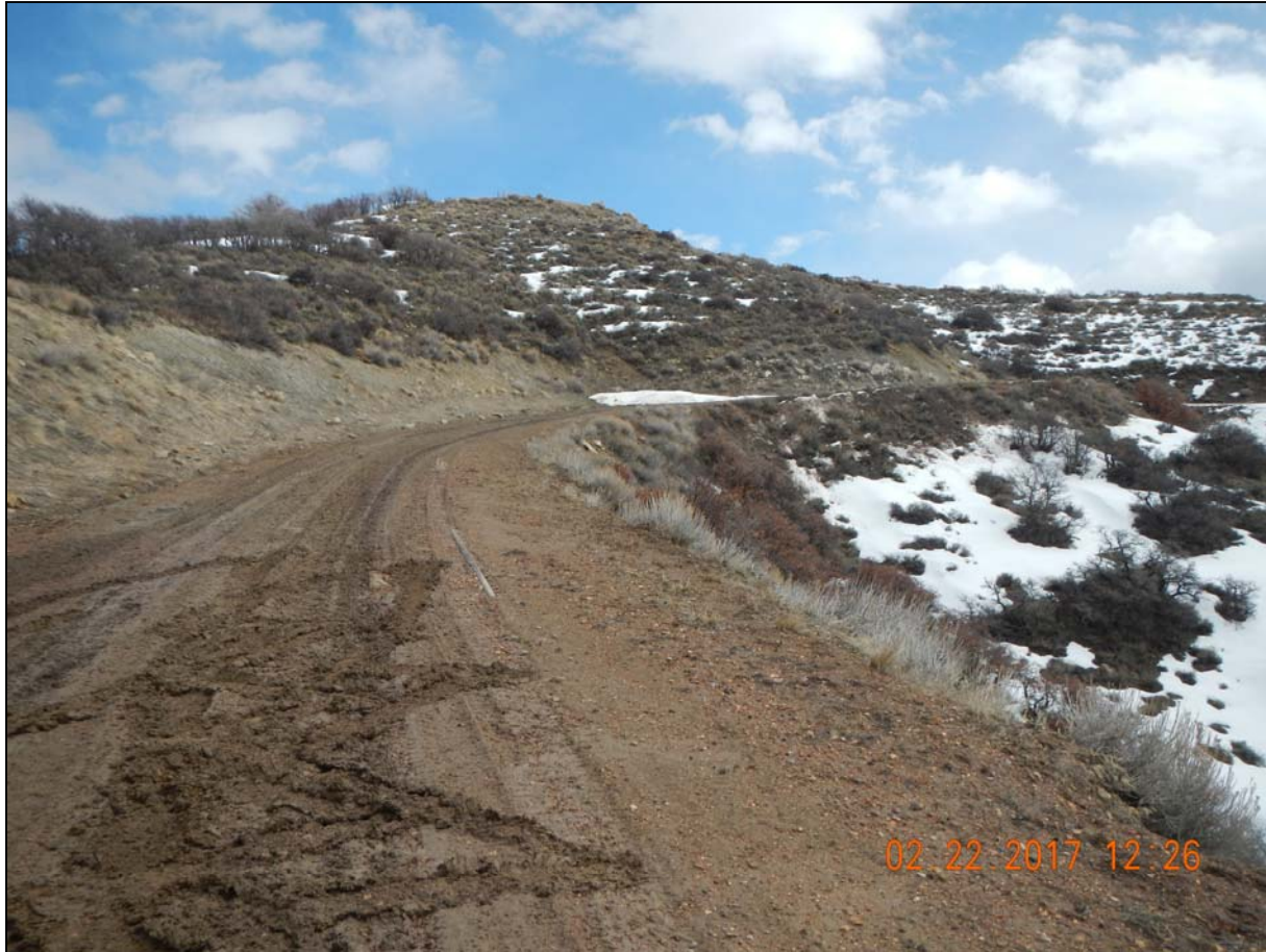
Photo 1. Photo on access road at point it became too muddy. (40.27658, -108.01469)
