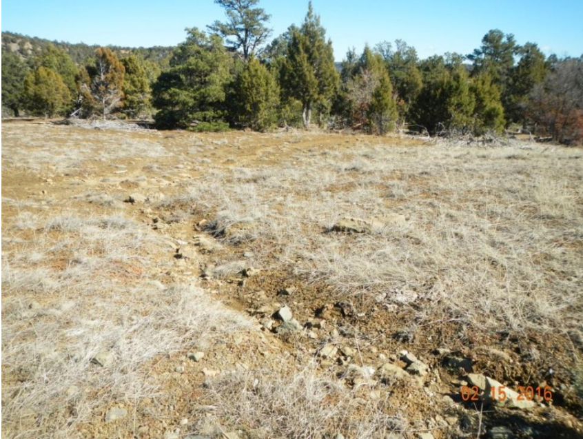
Photo 7: View of an erosional channel approximately 18 inches wide and 12 inches deep that is forming in the northeastern portion of the project area that needs stabilization.
