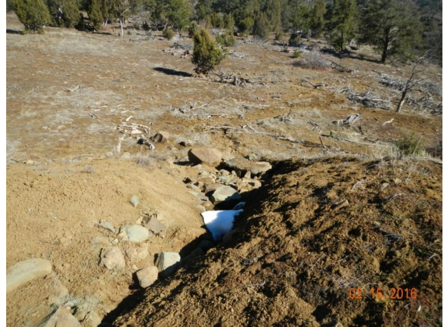
Photo 6: View of an erosional channel in the southeastern corner of the project area that needs stabilization measures.
