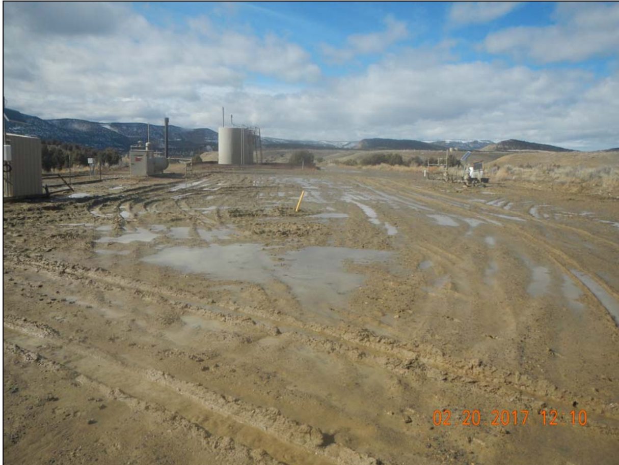
Photo 1. View at the entrance to location facing west.
