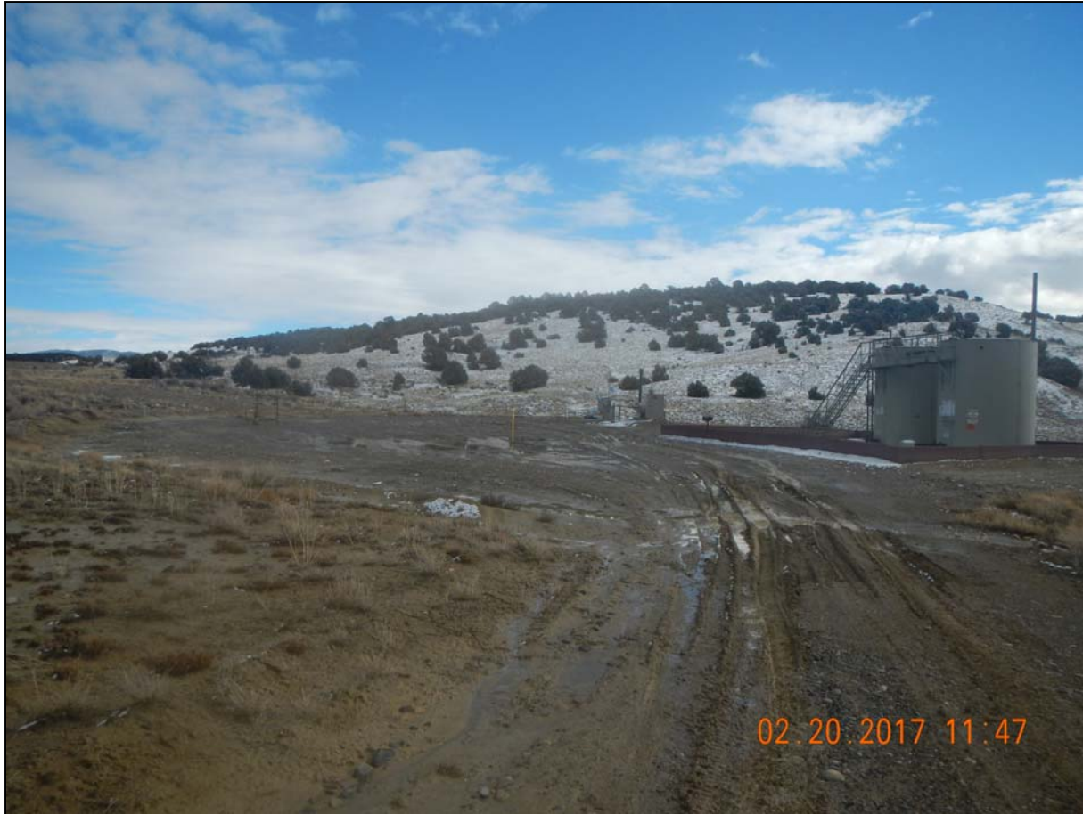
Photo 1. View at the entrance to location facing east.
