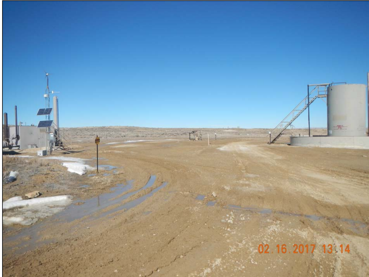
Photo 1. View of the location at the entrance facing north.
