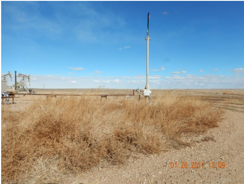
Photo 1. Photo taken 1/26/17 from the southern location, facing East, towards the flare. Kochia weeds next to the flare pose a fire hazard.
