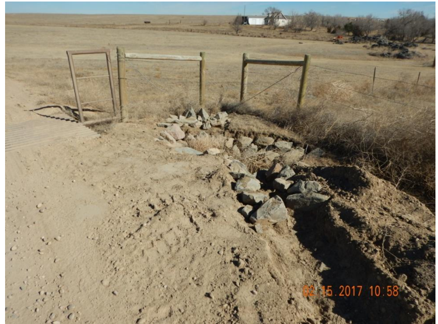
Photo 2. Photo taken from the entrance of location, facing North. Sediment trap has been installed along the east side of the access road.
