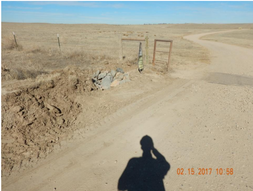
Photo 1. Photo taken from the entrance of location, facing North. Sediment trap has been installed along the west side of the access road.
