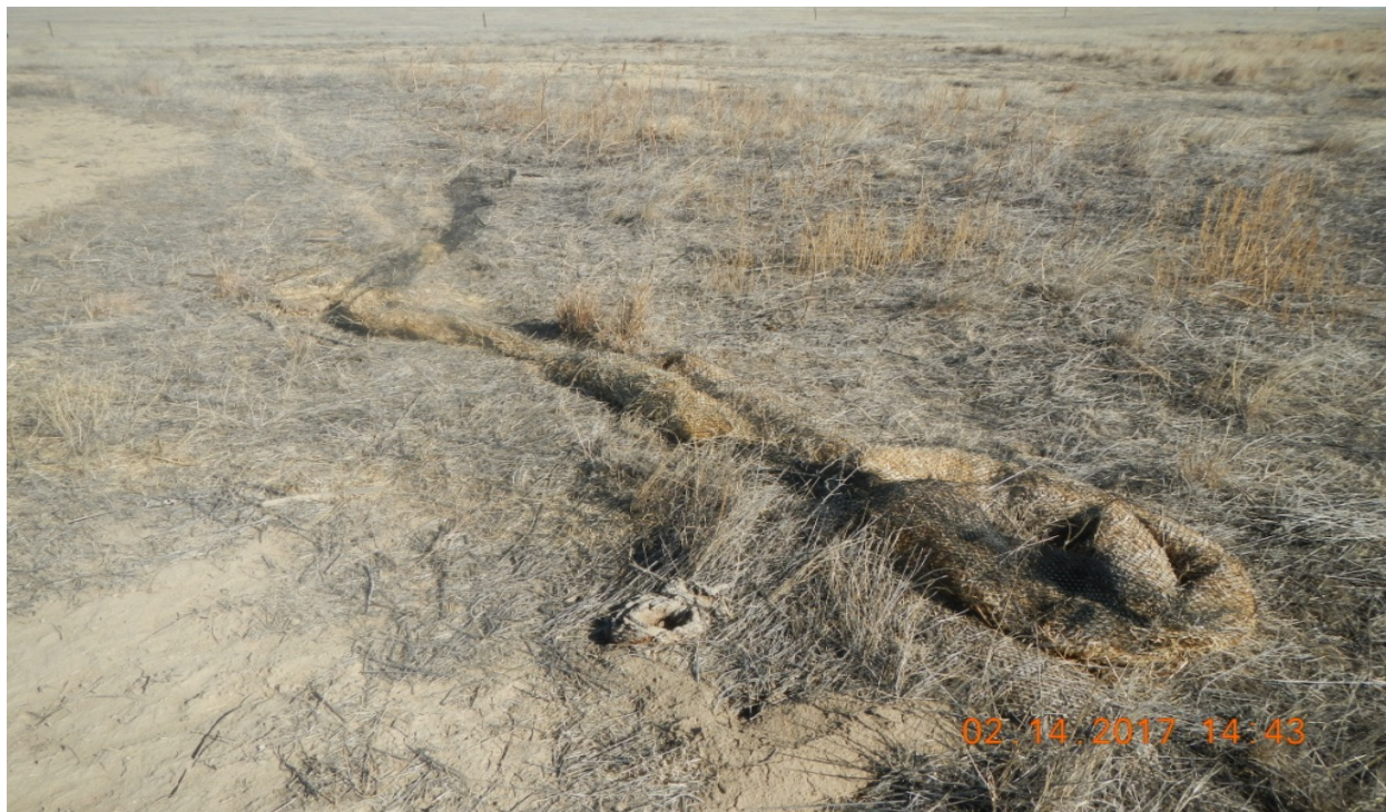
photo 3: There are degraded wattles that remains at the location.
