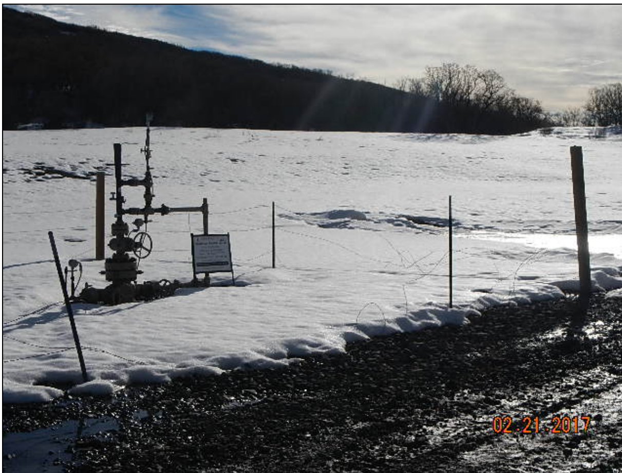
Photo 1. Wire fence is damaged. Potential wildlife or livestock hazard. Repair fence by 3/7/17.
