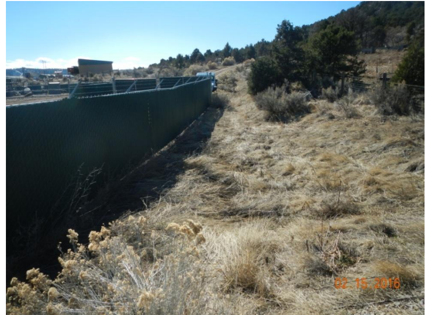
Photo 4. View of the western portion of the interim reclamation area. A vegetated silt trap is in good condition.
