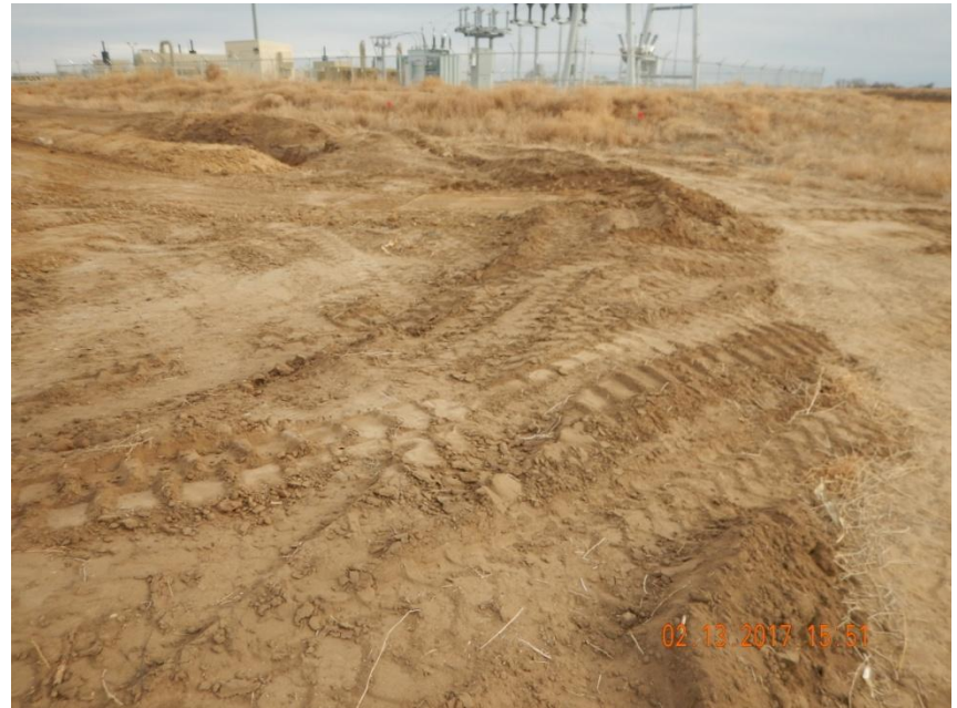
Photo 6. Photo taken from the southwest location, facing South. Ditch and berm BMPs appears to be damaged from equipment traffic. Need to repair BMP per Rule 1002.f.
