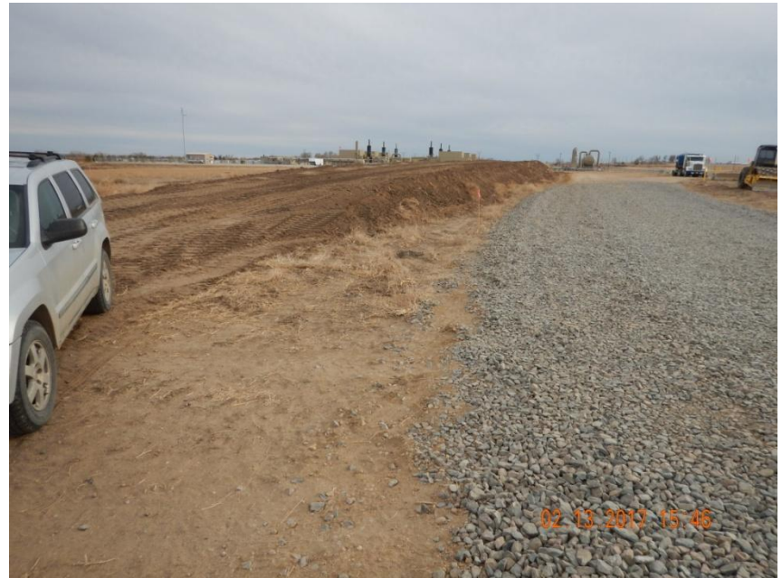
Photo 2. Photo taken from the northern location, facing South. Topsoil salvaged and stored along the eastern perimeter.
