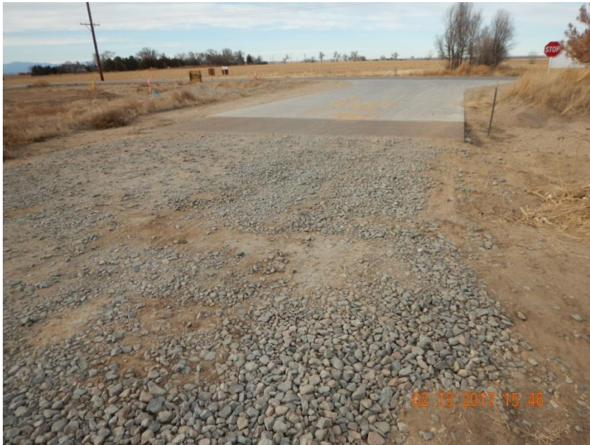
Photo 1. Photo taken from the entrance of location, facing North. Vehicle tracking pad installed with cattle guard. BMP appears to be properly functioning.
