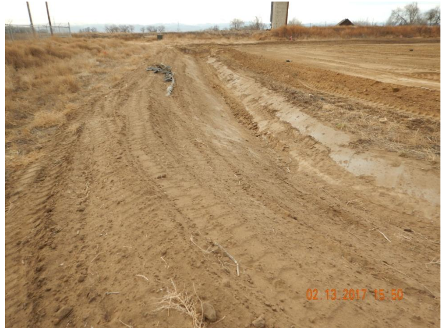
Photo 4. Photo taken from the southern location, facing West. Ditch and berm BMP installed around perimeter of location.
