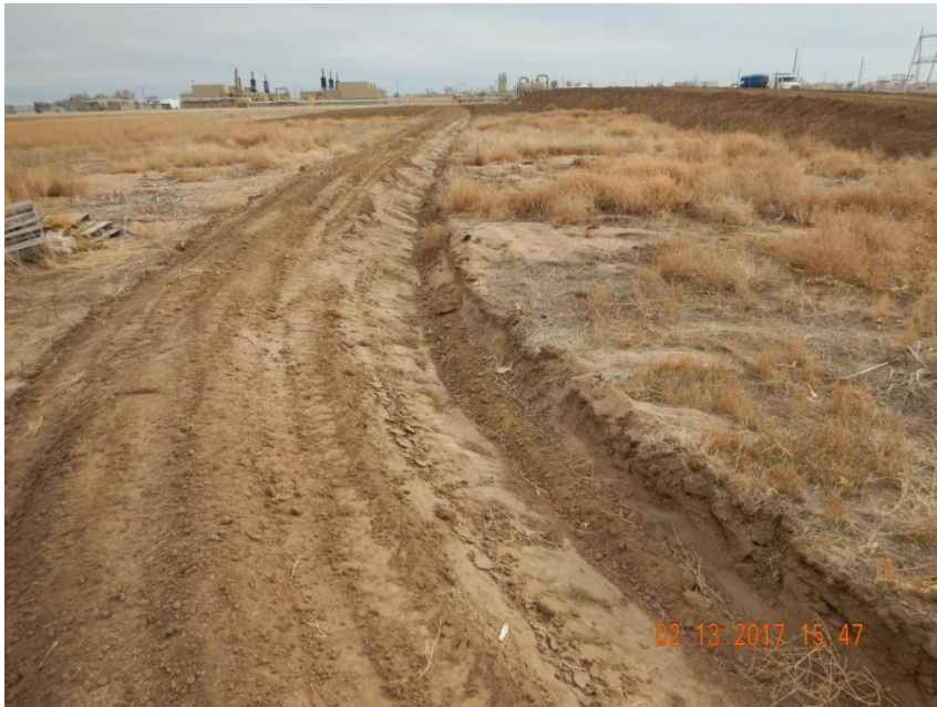
Photo 3. Photo taken from the northeast location, facing South. Ditch and berm BMP installed around perimeter of location.
