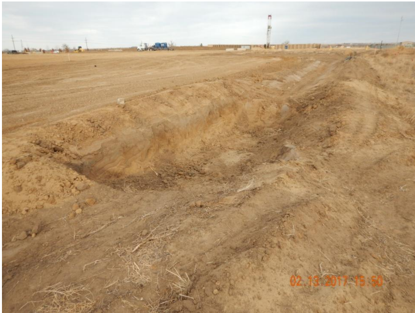
Photo 5. Photo taken from the southwest location, facing East. Sediment trap is IN-PROCESS of being constructed.
