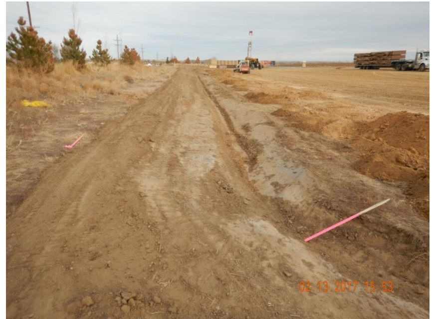
Photo 8. Photo taken from the northwest location, facing East. Ditch and berm BMP installed along perimeter of location.
