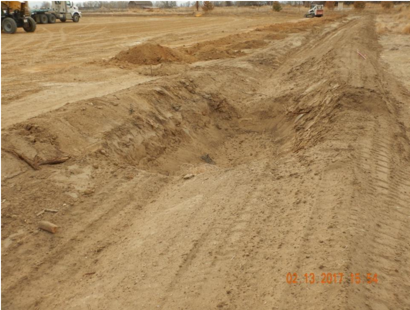
Photo 9. Photo taken from the northern location, facing West. Sediment trap is IN-PROCESS of being constructed.
