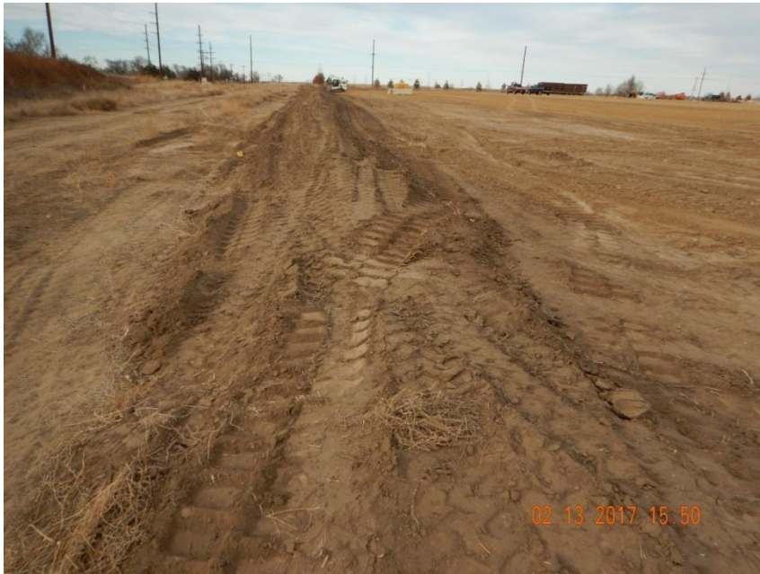
Photo 7. Photo taken from the southwest location, facing North. Ditch and berm BMP installed along perimeter of location. Ensure all portions of the berm are properly compacted to manage pollutant contributions to stormwater runoff from unconsolidated soil material.
