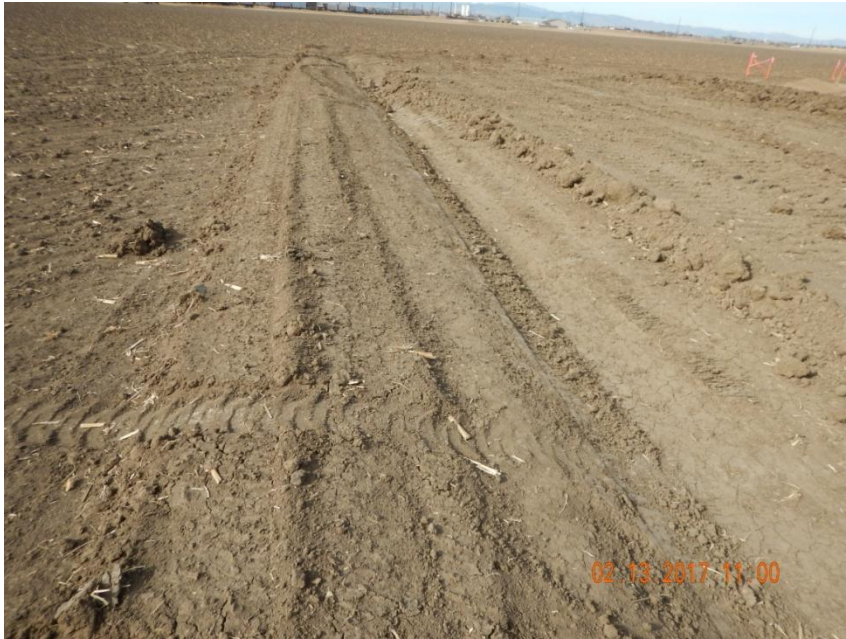
Photo 5. Photo taken from the western location, facing West. Ditch and berm BMP installed around the perimeter of location. Equipment traffic should stay off BMPs to ensure BMP is not damaged so BMP properly functions.
