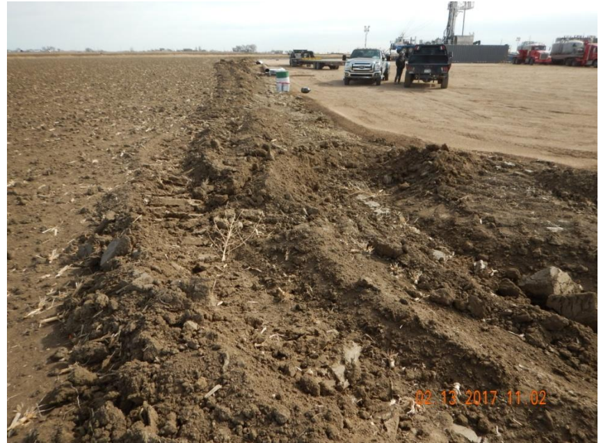
Photo 8. Photo taken from the northwest location, facing East. Berm has not been compacted leaving excessive soil material unconsolidated.
