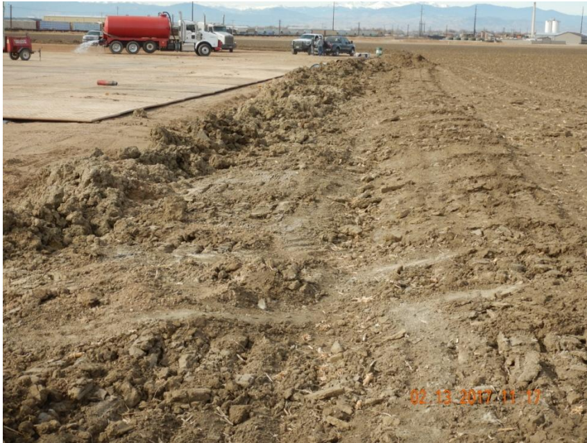
Photo 9. Photo taken from the northeast location, facing West. Excessive, unconsolidated soil material along the ditch BMP.
