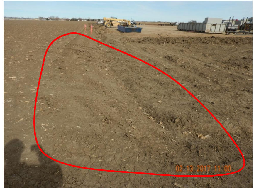
Photo 6. Photo taken from the western location, facing North. BMP may need to be re-installed because equipment traffic has damaged the BMP. Equipment traffic should stay off BMPs to ensure BMP is not damaged so BMP properly functions.
