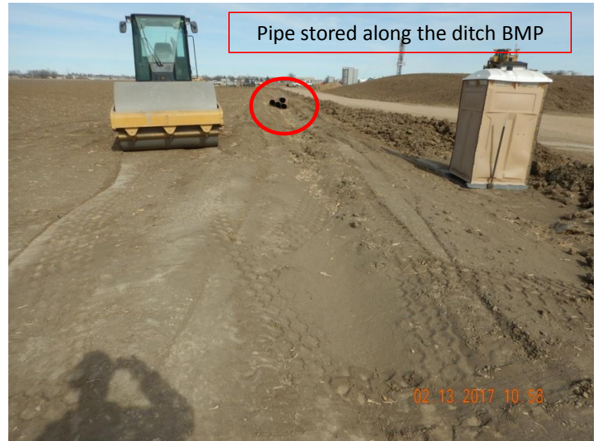
Photo 4. Photo taken from the southwest location, facing North. Ditch and berm BMP installed around the perimeter of location. Berm may need to be built to a sufficient height as the height appears minimal along portions of the BMP. Also, keep equipment and debris free of the BMP.
