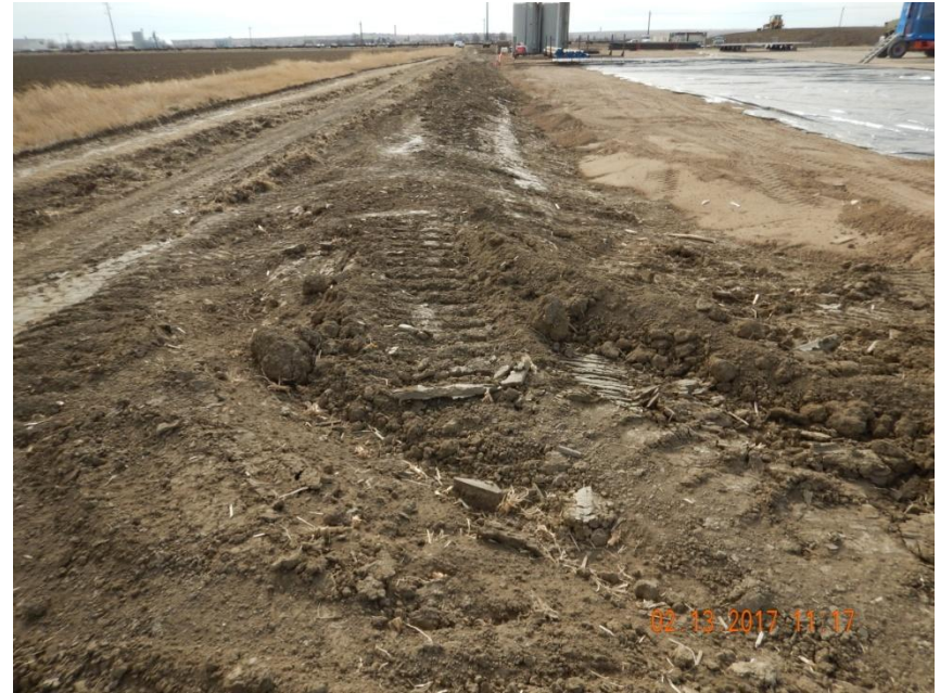
Photo 10. Photo taken from the northeast location, facing South. Ditch and berm BMP installed around the perimeter of location. Unconsolidated soil material along the ditch BMP shall be compacted.
