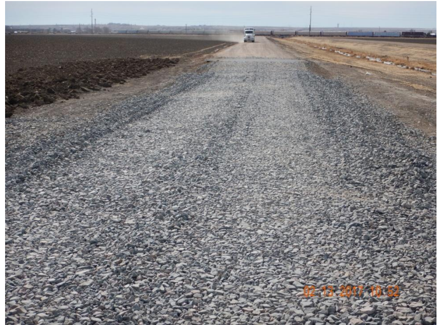
Photo 2. Photo taken from the entrance of location, facing South. Vehicle tracking pad installed and properly functioning. In addition, two (2) cattle guards have been installed.
