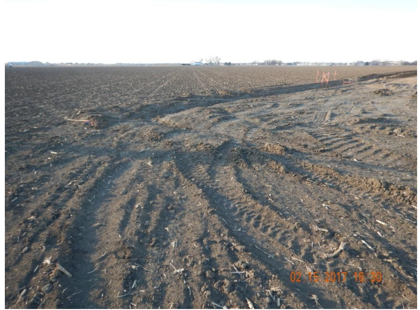
Photo 14. Photo taken on 2/15/17 from the western location, facing Northwest. BMP may need to be re-installed because equipment traffic has damaged the BMP. Equipment traffic should stay off BMPs to ensure BMP is not damaged so BMP properly functions.
