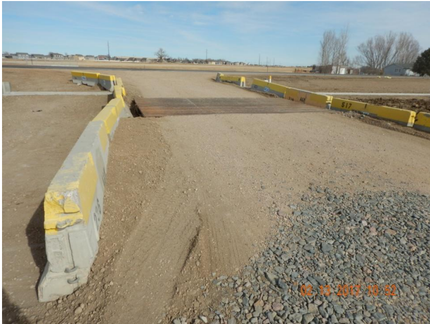
Photo 1. Photo taken from the entrance of location, facing North. Vehicle tracking pad installed and properly functioning. In addition, two (2) cattle guards have been installed.
