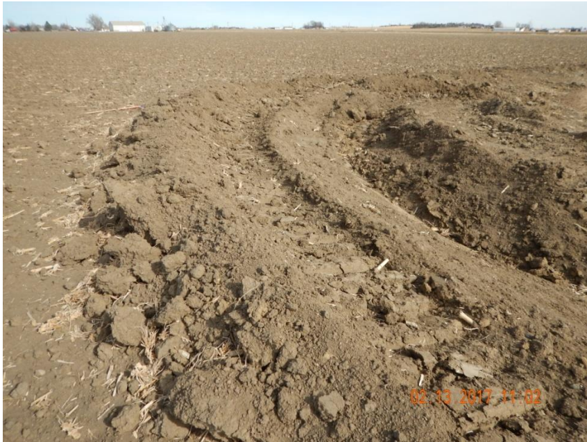
Photo 7. Photo taken from the northwest location, facing Northeast. Berm has not been compacted leaving excessive soil material unconsolidated.
