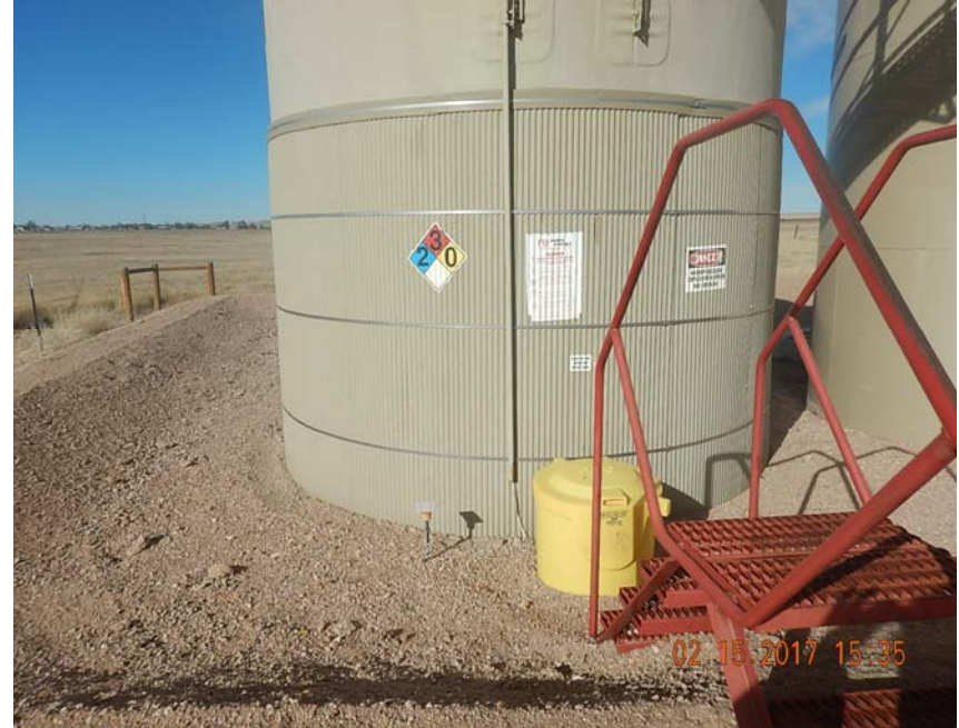
Photo 1: No contents, capacity on production tank
