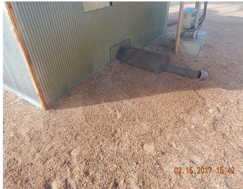
Photo 3: Stained soil at exhaust
