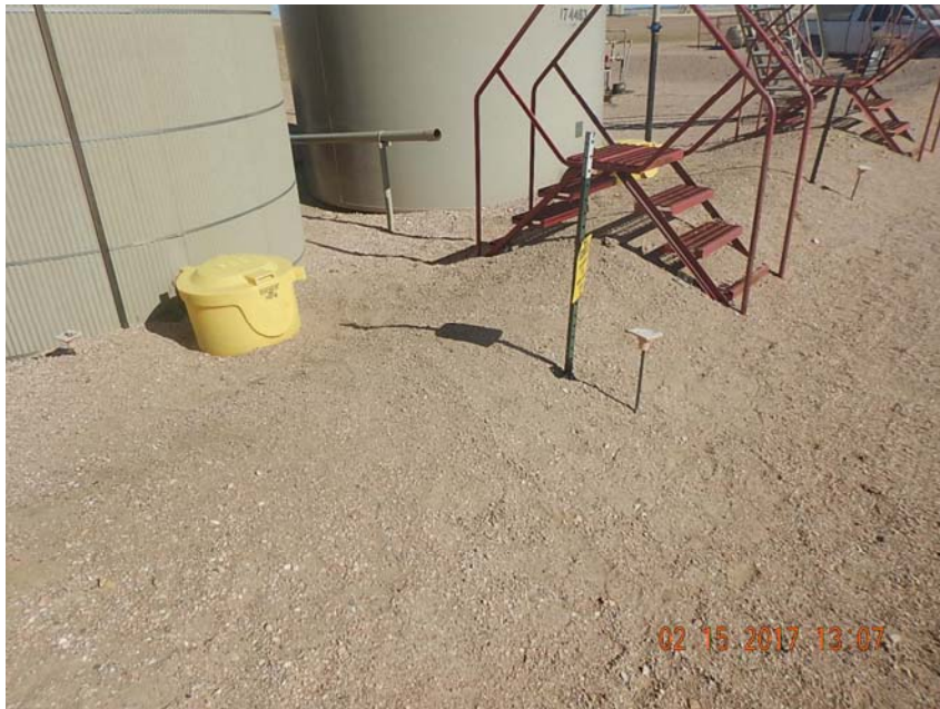
Photo 4: Low berms at loadout valve
