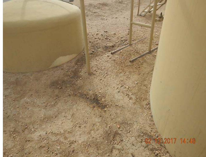
Photo 5: Stained soil at produced water tank
