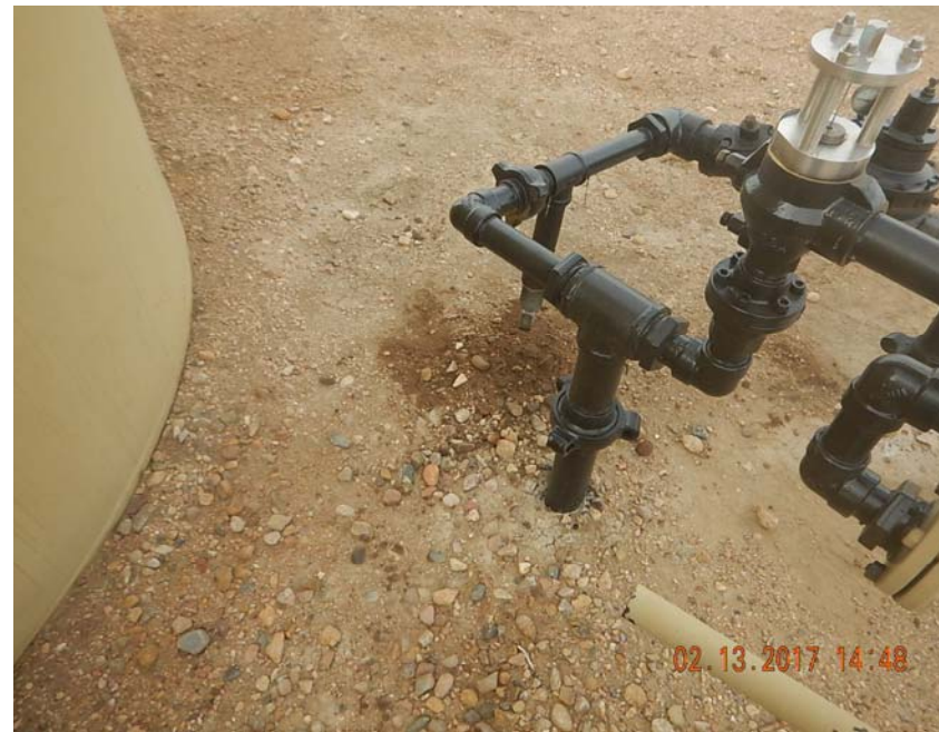
Photo 2: Stained soil around tank
