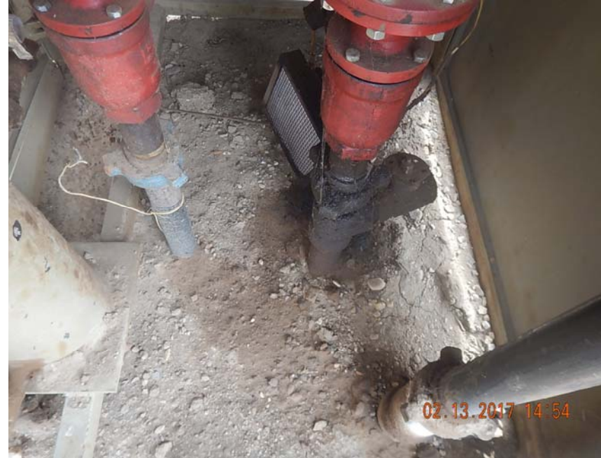
Photo 8: Stained soil in separator house
