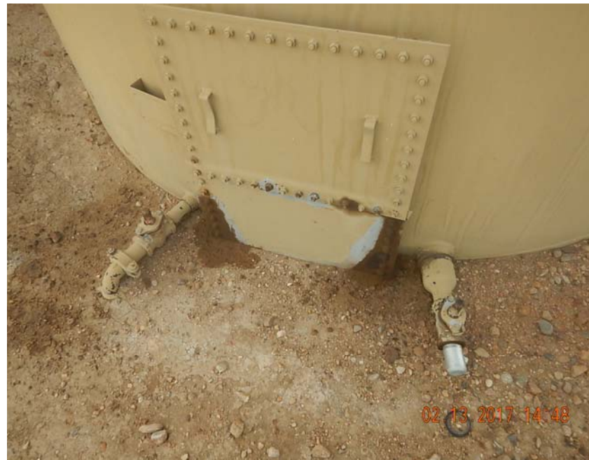
Photo 3: Stained soil at hatch
