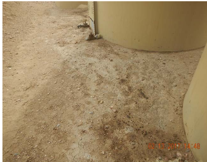
Photo 4: stained soil between tanks
