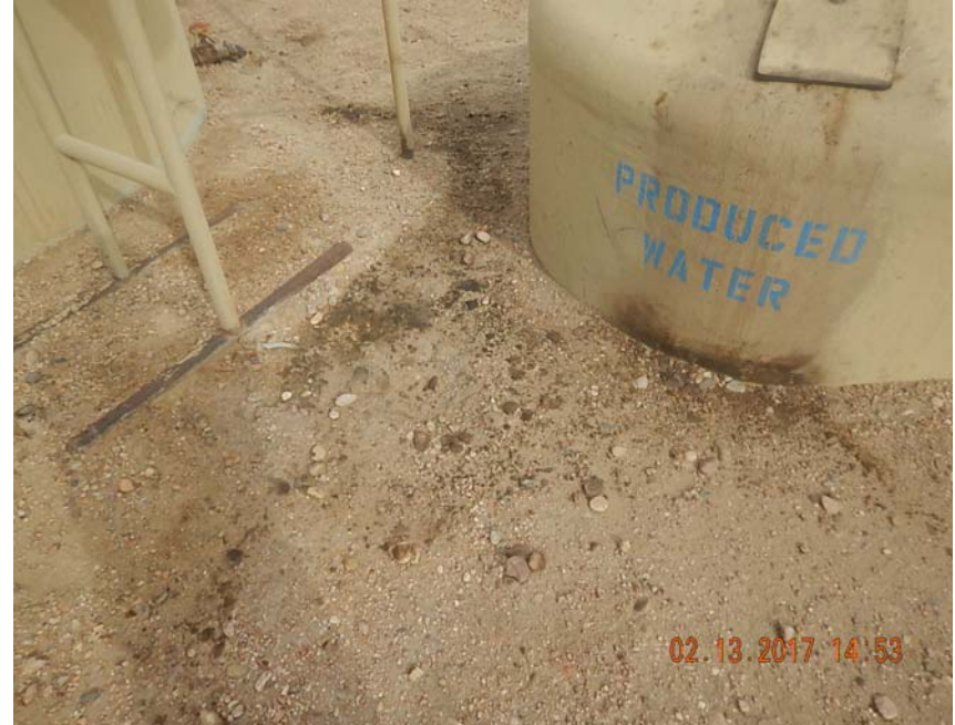
Photo 6: Stained soil at produced water tank
