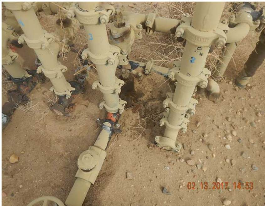
Photo 9: Stained soil at manifold
