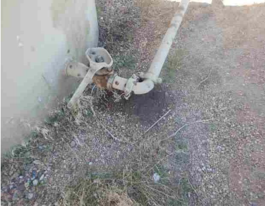
Prior inspection photo for comparison purposes only
