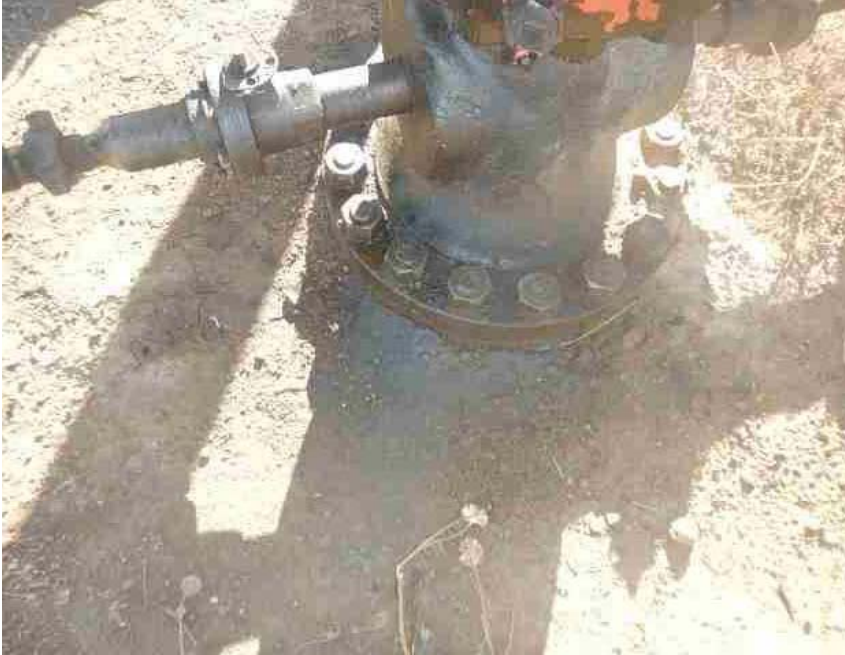
Prior inspection photo for comparison purposes only
