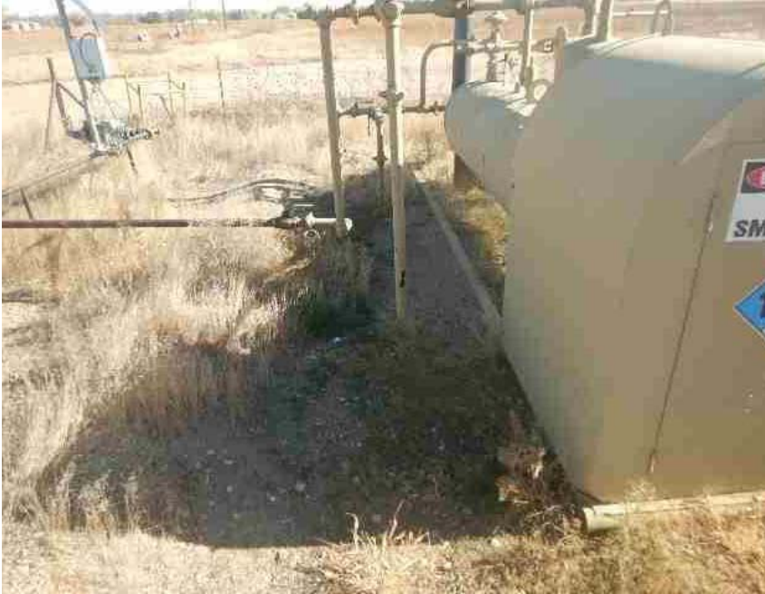
Prior inspection photo for comparison purposes only
