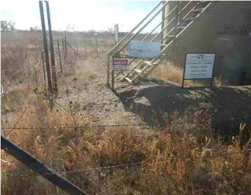
Prior inspection photo for comparison purposes only
