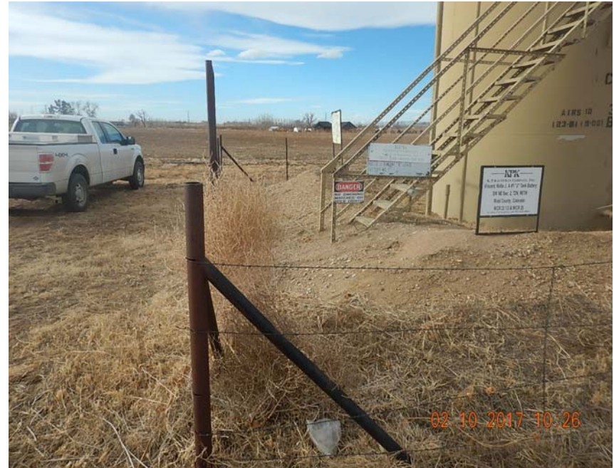
Photo 2: Weeds controlled at tank battery, looking S
