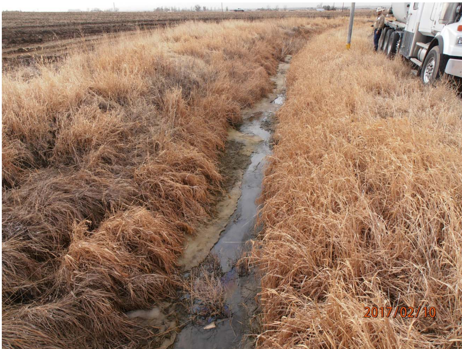
Vacuum truck preparing to recover free liquid hydrocarbons and surface water exhibiting visual impacts, stationed approximately 400 feet downgradient of release point. Photo is looking south and downgradient.
