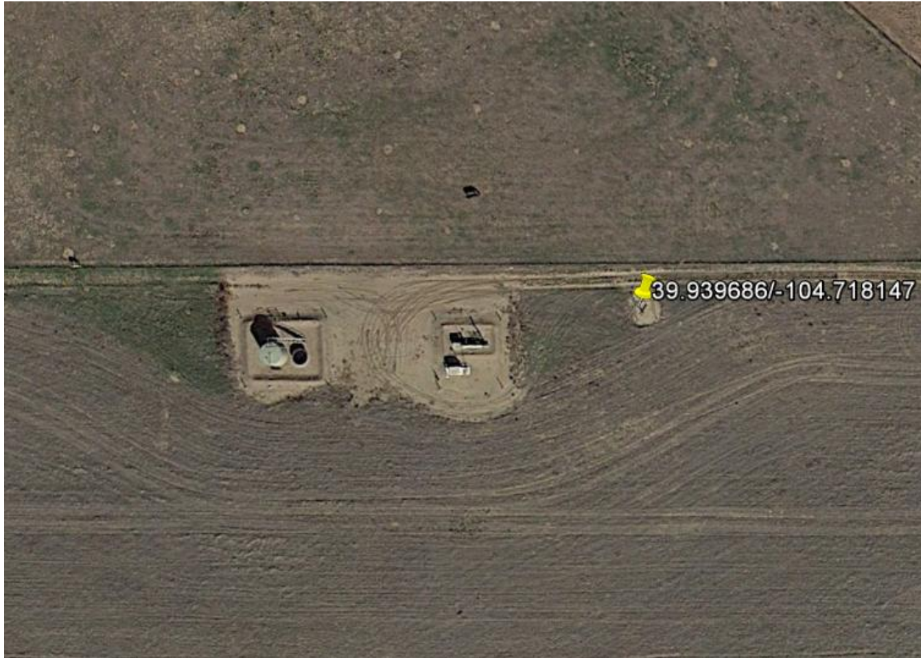
Google Earth aerial imagery taken October 7, 2012 of the well and tank battery location while it was active.
